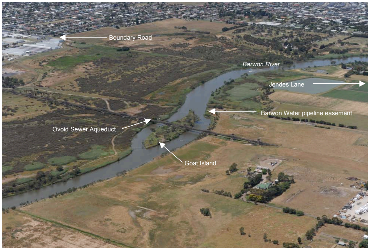
Photo 2 - North East Industrial Precinct view north east from Kings Lane to the Ovoid Sewer Aqueduct Source: Parks Victoria July 2010
