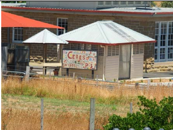
Photo 4: Early timber shelter shed, north & east elevations, 2017.
