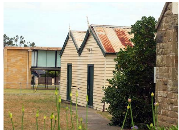
Photo 3: Former Sunday School, east elevation, 2016. Source: David Rowe.
