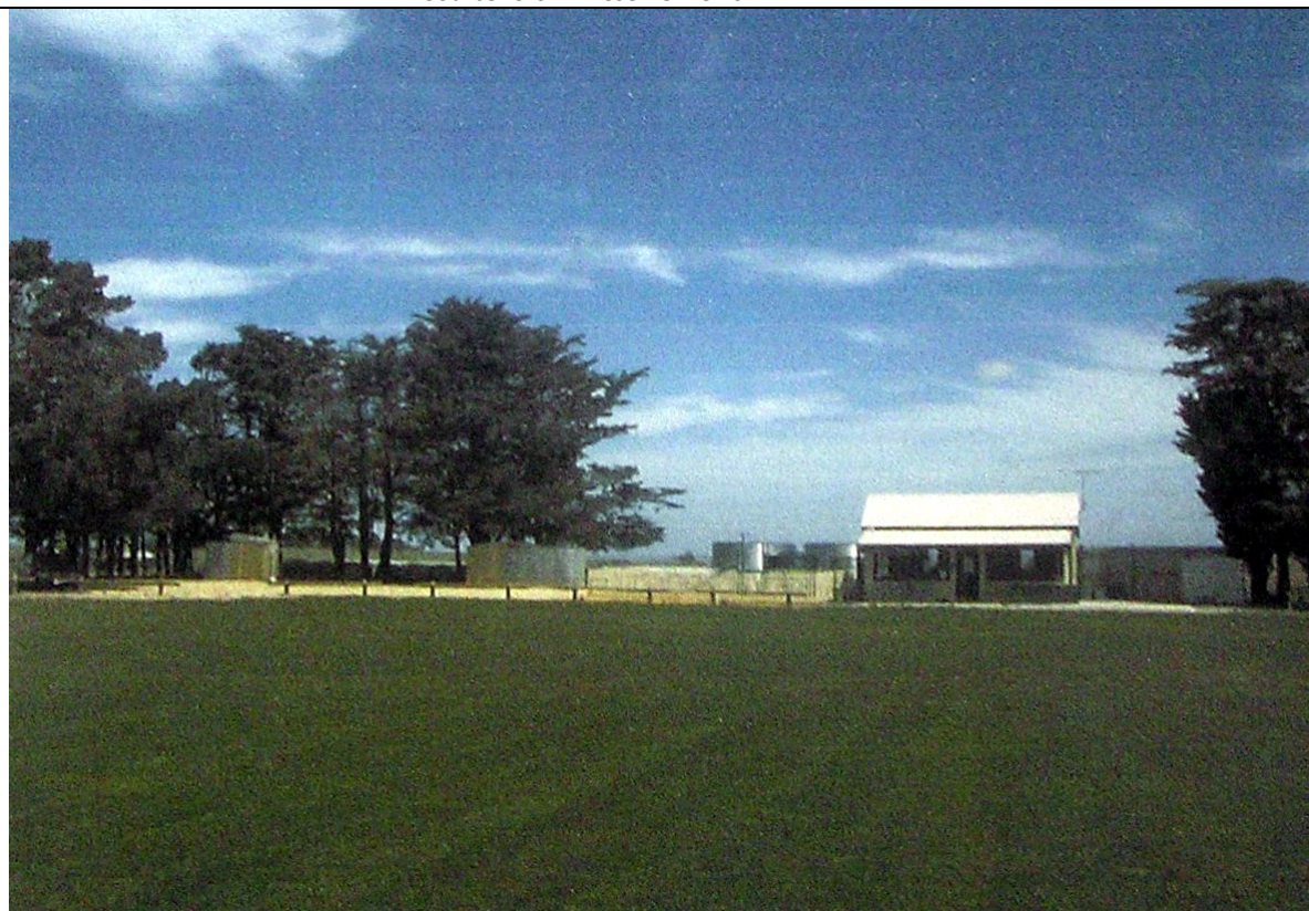
Figure 9: Ceres Recreation Reserve looking south to the pavilion following alterations, n.d. [c.2014]. Source: Crown Reserve file Rs 4144 DELWP.
