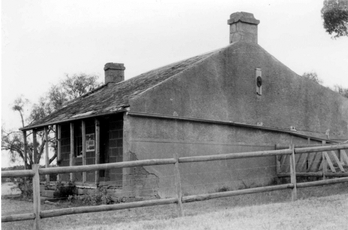
Figure 5: J.T. Collins, 'Barwonside', front and south elevations, c.1980-85. Source: La Trobe Picture collection, State Library of Victoria, accession H94.200/650.
