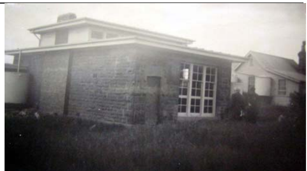
Figure 15: Newly completed Ceres School (south & west elevations), 1950. Source: VPRS 10516/P3 Unit 7 Public Record Office Victoria.
