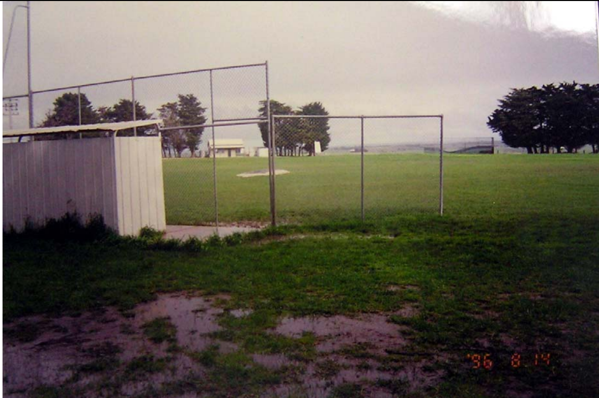
Figure 8: Ceres Recreation Reserve looking south to the pavilion prior to alterations & additions, 14 August 1996. Source: Crown Reserve file Rs 4144 DELWP.
