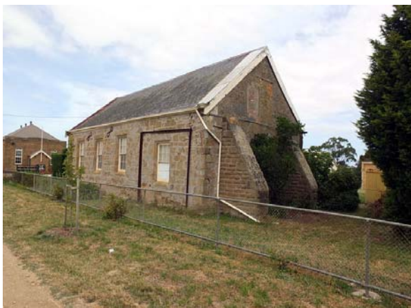
Photo 2: Former Church building, north & west elevations, 2016. Source: David Rowe.
