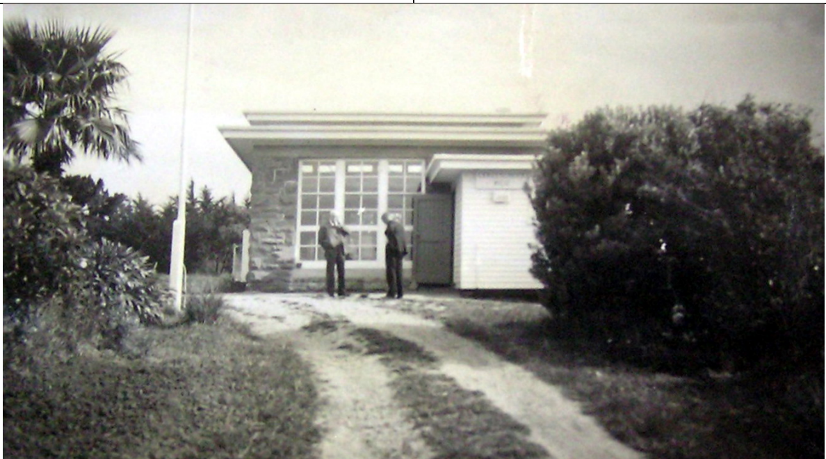
Figure 13: Newly completed Ceres School (front elevation), 1950.
