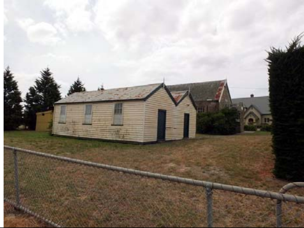
Photo 4: Former Sunday School (middle ground) & Church (background), south elevations, 2016.
