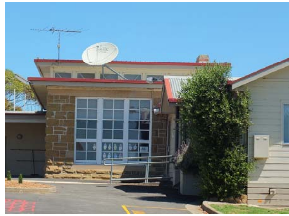
Photo 3: Detail of front elevation of the old Ceres Primary School building, 2017.
