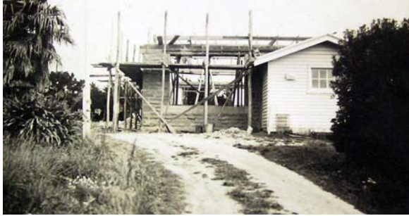
Figure 11: Ceres School under construction (front/north elevation), 15 Sept 1950.
