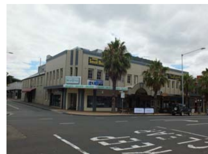
Former Sparrow Building, 54-58 Moorabool St, 2016. Source: David Rowe.
