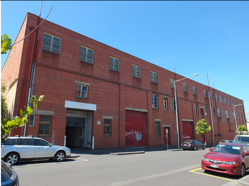
Photo 3: Former Woolstore, south elevation, looking east, 2015.
