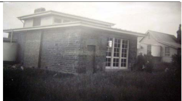
Figure 15: Newly completed Ceres School (south & west elevations), 1950. Source: VPRS 10516/P3 Unit 7 Public Record Office Victoria.
