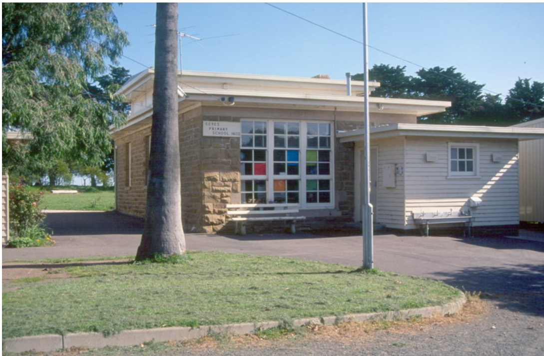
Figure 17 Ceres Primary School, front elevation, c.1993 Source: Late Ian Wynd photograph collection.
