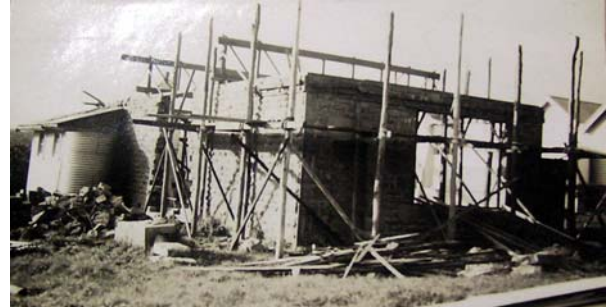
Figure 12: Ceres School under construction (south & west elevations), 15 Sept 1950. Source: VPRS 10516/P3 Unit 7 Public Record Office Victoria.
