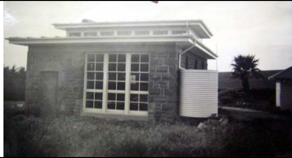
Figure 16: Newly completed Ceres School (south elevation) 1950. Source: VPRS 10516/P3 Unit 7 Public Record Office Victoria
