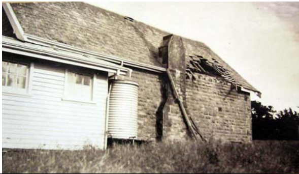
Figure 6: West view of Ceres State School showing roof damage, 6 December 1948.
