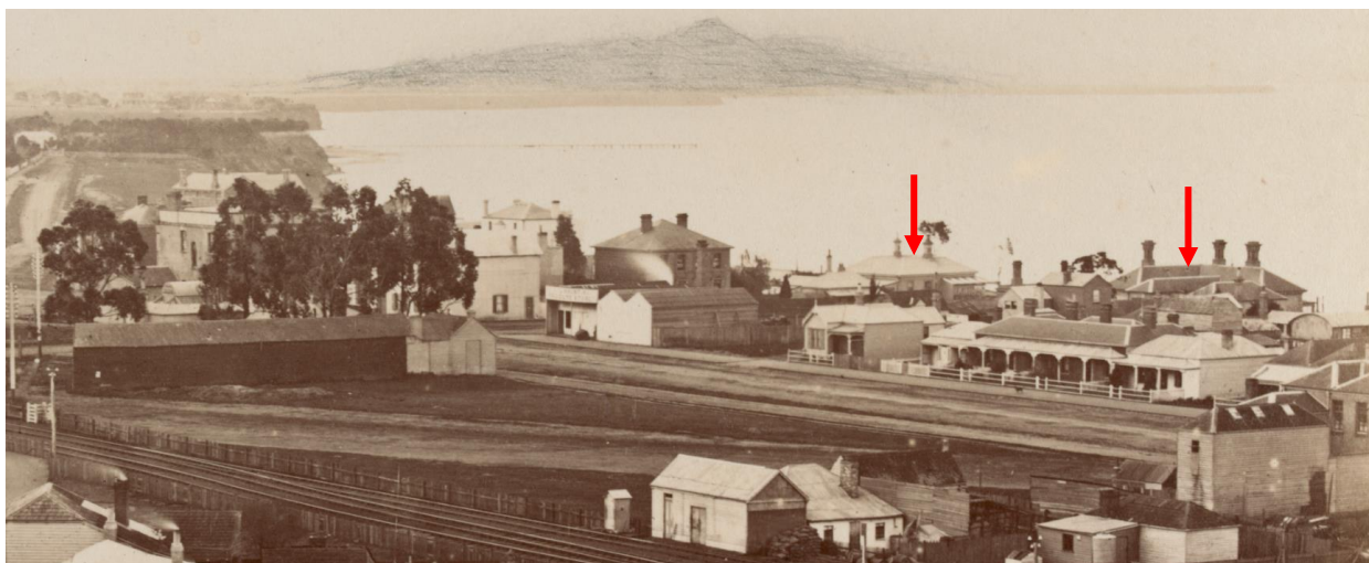
'View of Corio Bay, from St. Paul's Tower, Geelong' (Fred Kruger, circa 1882)
