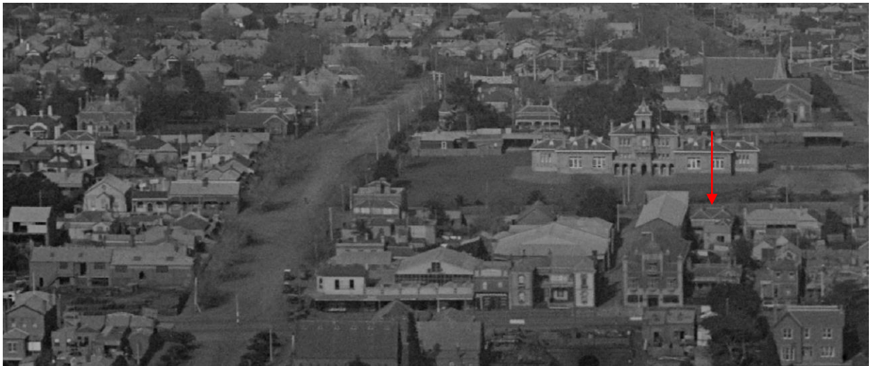
'Rail yards and Geelong Railway Station' (circa 1926, C D Pratt) Looking south, the subject site is indicated (Source: State Library of Victoria H91.160/677)
