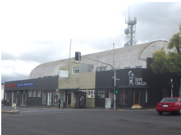
Ryrie Street, north-west corner
