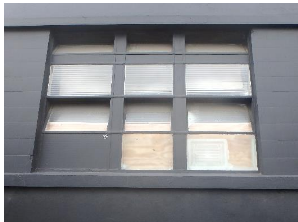
Original window, Ryrie Street
