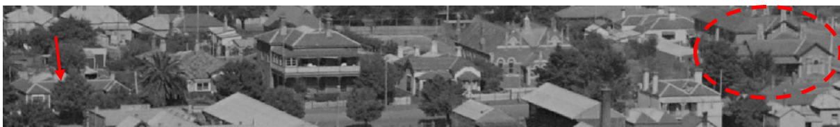
'Geelong' (C Pratt, March 1938) Showing Myers Street, between Gheringhap Street and Fenwick Street – nos 38+40 (left/arrow) and no. 20 (right/circle) (Source: SLV, H91.160/632)
