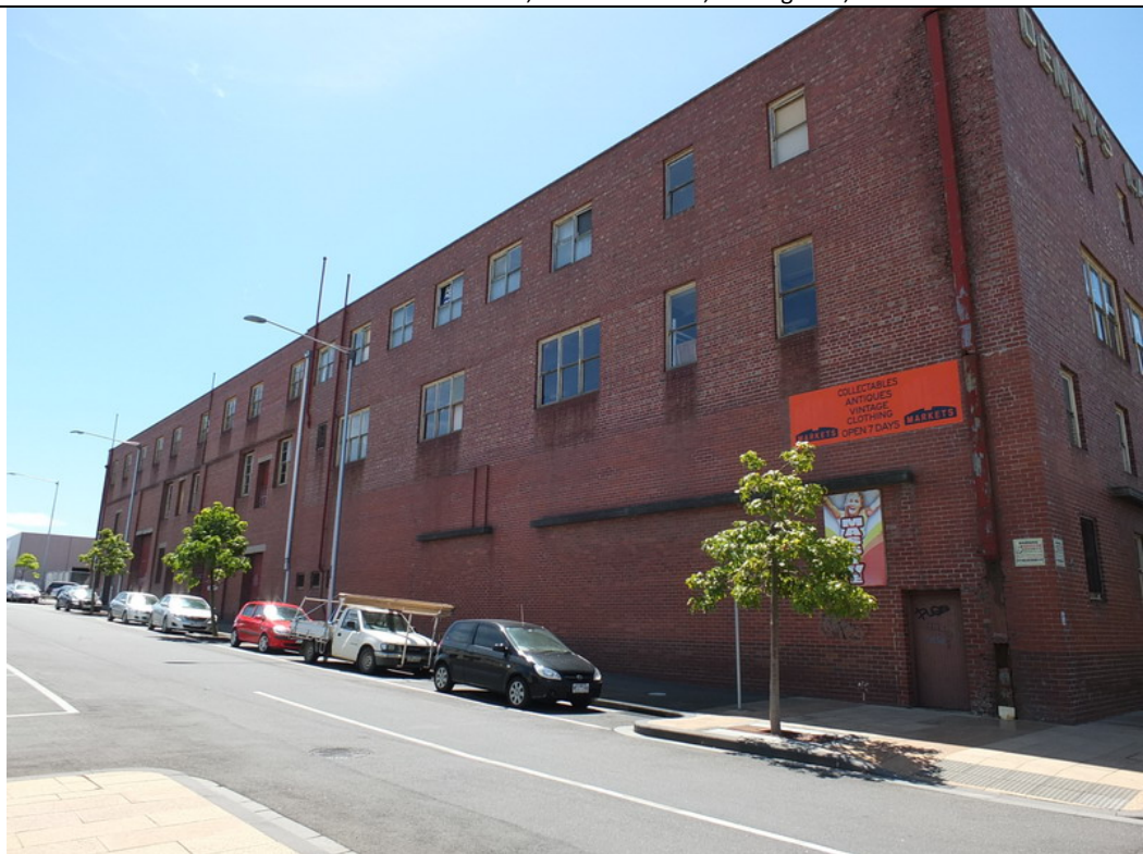
Photo 4: Former woolstore, south elevation, looking west, 2015.
