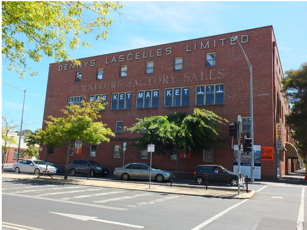
Photo 5: Former Woolstore, east elevation, 2015.
