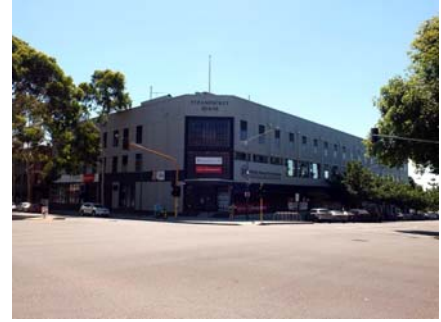
Former woolstore (Steampacket House), 6-24 Moorabool St, 2017. Source: David Rowe.
