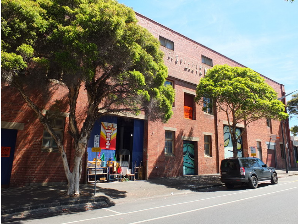
Photo 2: Former woolstore, north elevation (original portion of 1919), 2015.
