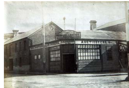
Sparrow Building, 58 Moorabool St, before 1932 (the gabled building at the rear is the original building). Source: Holmes photograph collection, c/o David Rowe.
