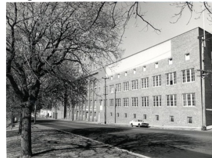
Western and central portions of the former woolstores complex, Western Beach Road, showing alterations and additions, including the construction of the upper floor to the corner bay and the 1940s windows. Source: Ian Wynd collection.
