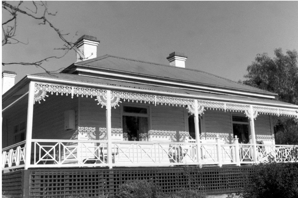
Figure 5: 'Erinvale', 285 Gully Road, 1997. Source: David Rowe.
