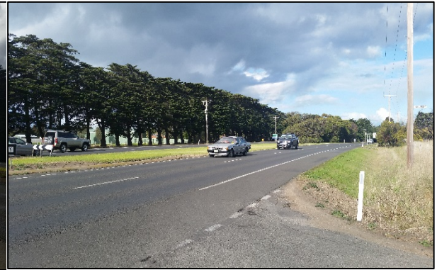
Figure 10: Bellarine Highway – View East
