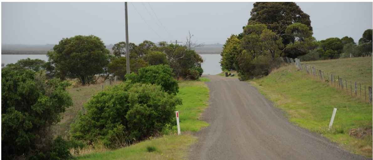
Figure 8 Mollers Lane looking south
