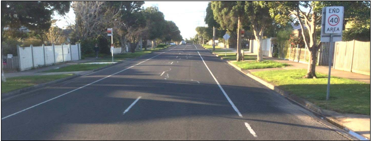
Figure 2.8 Ash Road (facing north from Lawrence Street)
