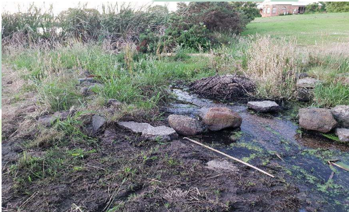
Plate 3. Water flowing over the dam wall into the drainage line
