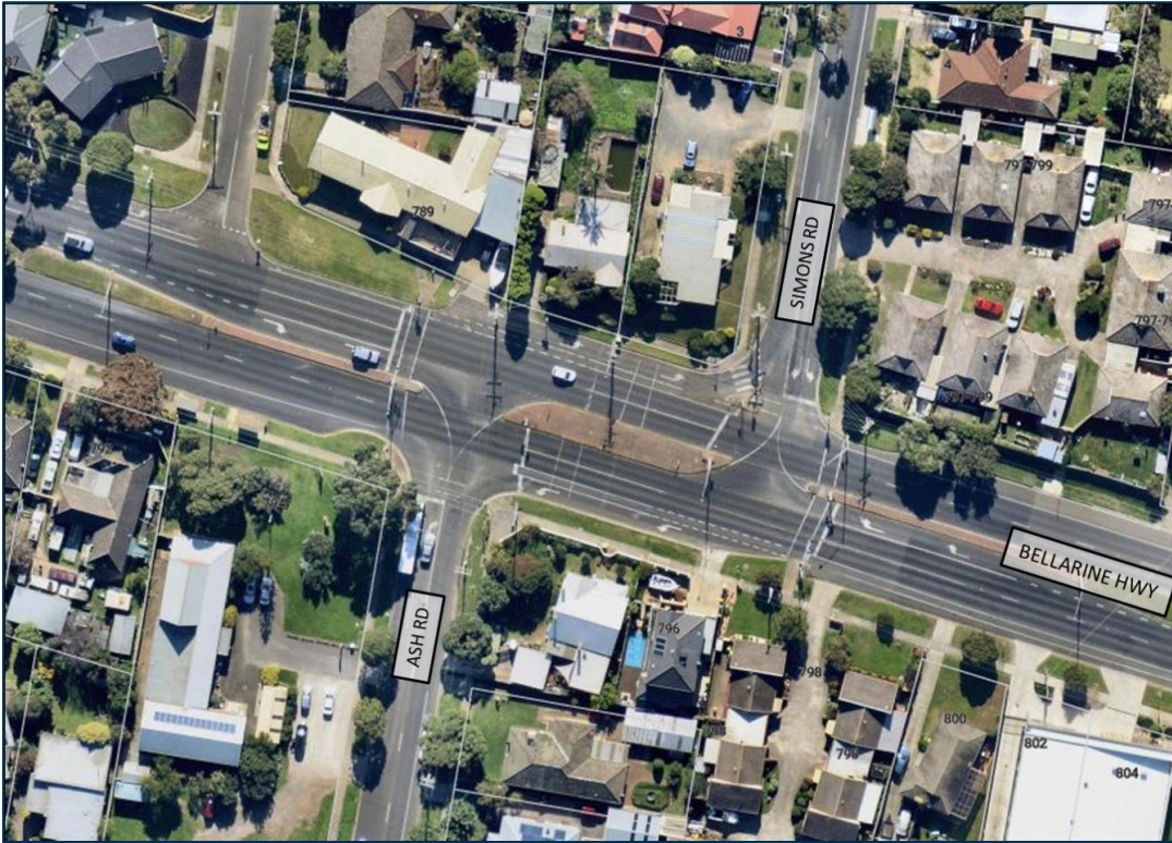
Figure 2-5 Bellarine Highway / Ash Road Intersection
