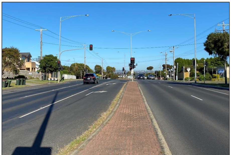
Figure 5-3: Bellarine Highway – looking west towards Simons Road / Ash Road
