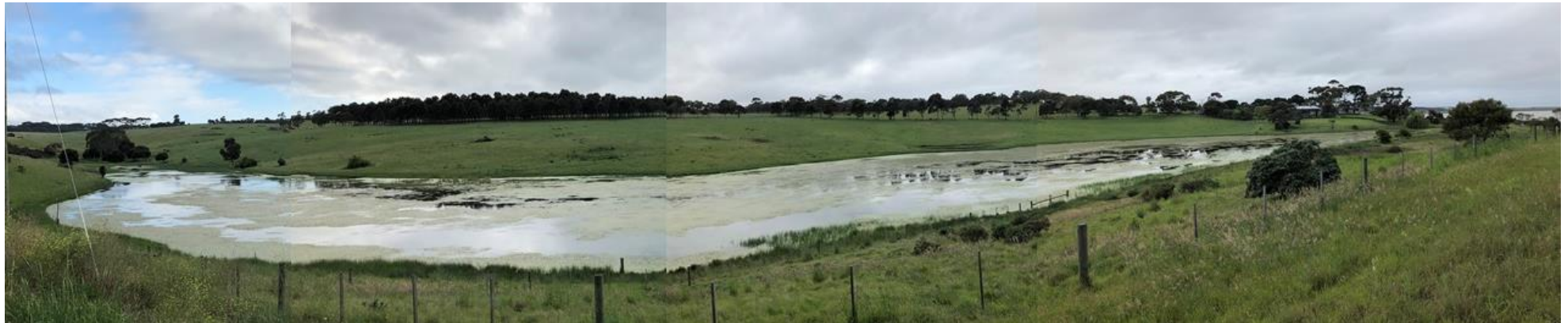
Photo 4 – Panorama View from Mollers Lane over dam at end of catchment, significant algae observed on surface, indicative of poor water quality
