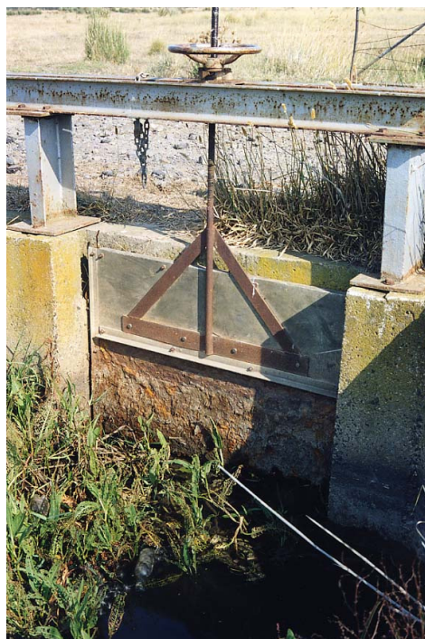
Figure 2-4 Hospital Swamp Inlet Regulator Structure
