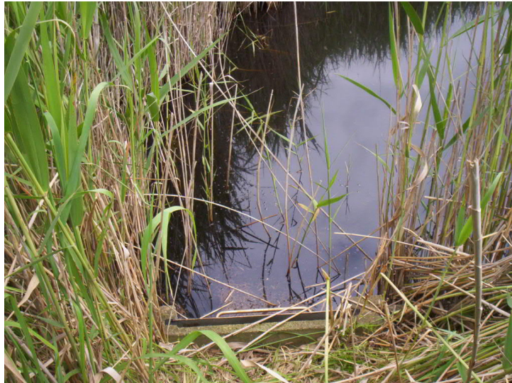
Figure 2-5 Hospital Swamp Outlet Regulator Structure
