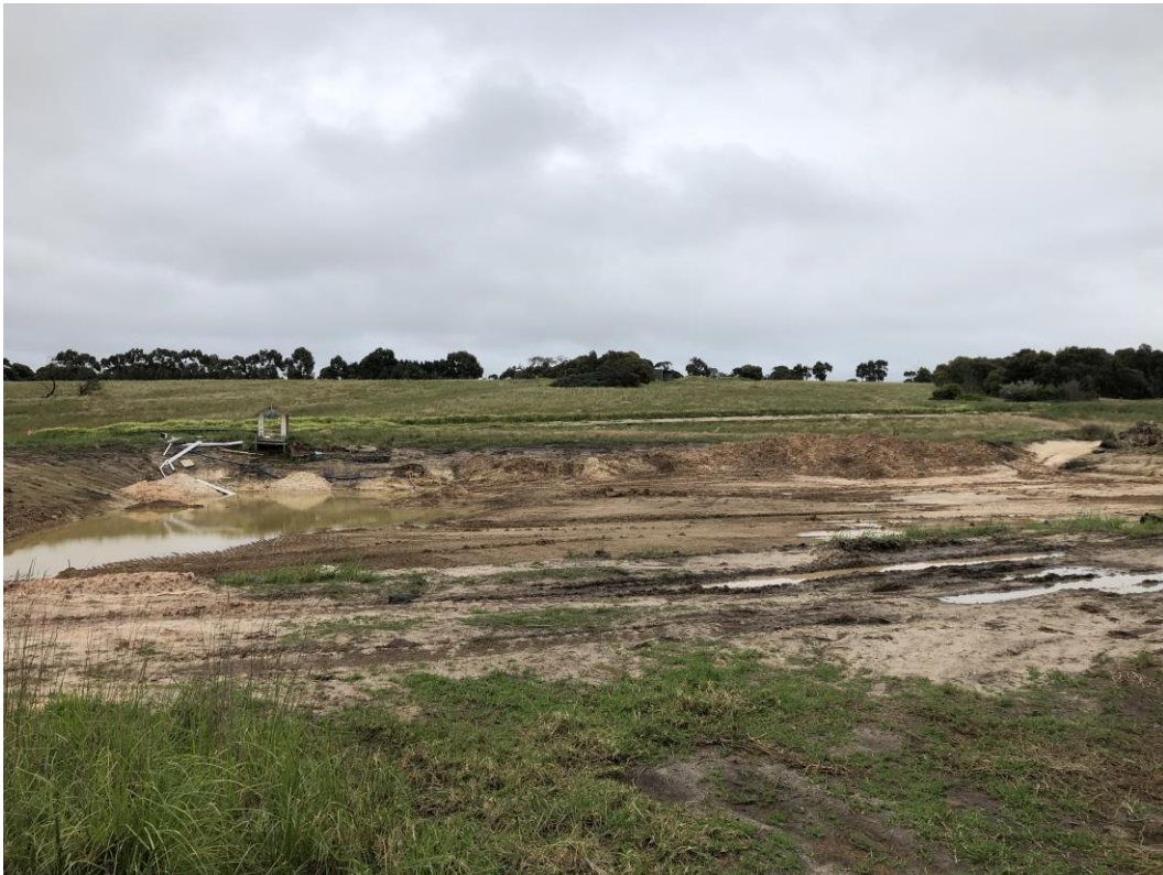
Photo 13 – View west from Mollers Lane at Tributary 1 dam decommissioning works.
