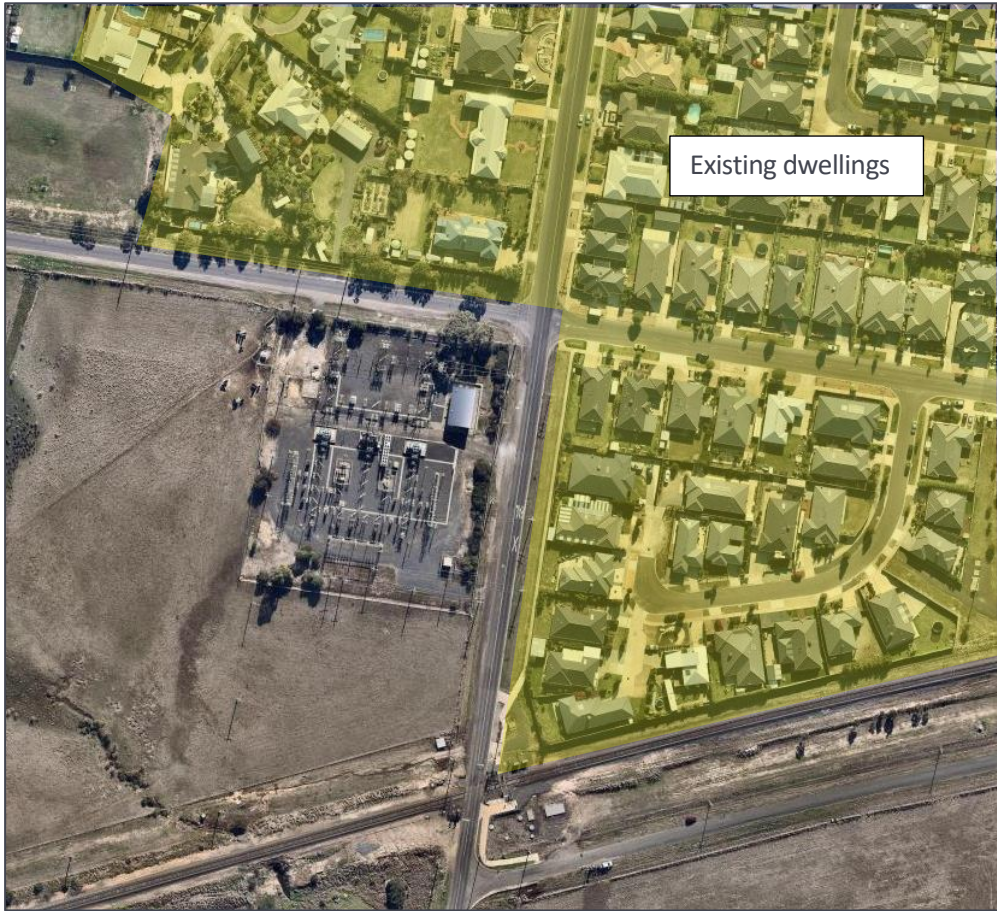
Figure 3: Existing dwellings close to substation site
