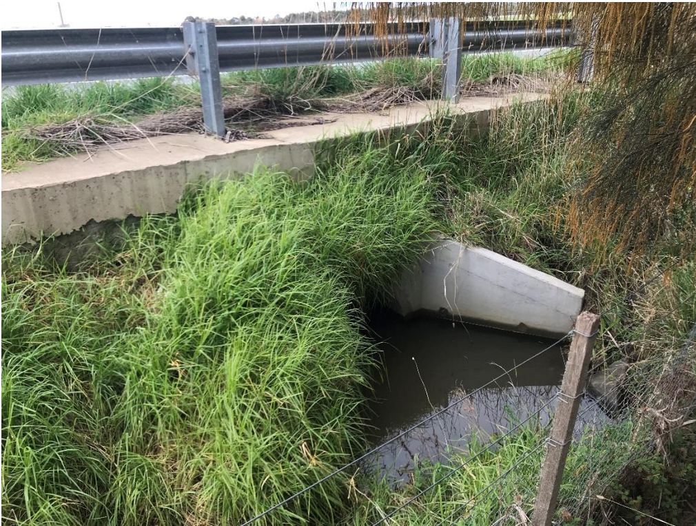
Existing Ghazeepore Rd culvert
