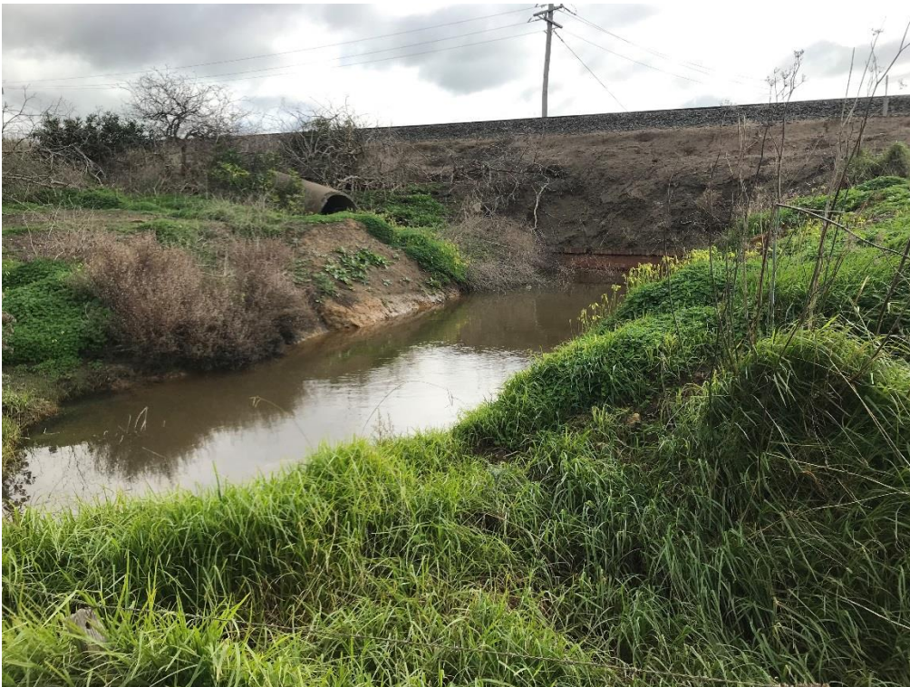
Existing Warrnambool - Geelong railway Culvert submerged (downstream)
