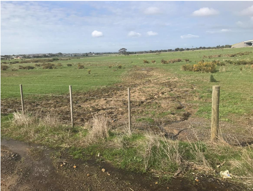
Erosion within the upstream end of site (looking east)
