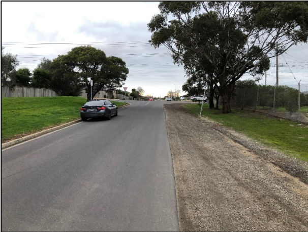
Figure 5: Hams Road – View east
