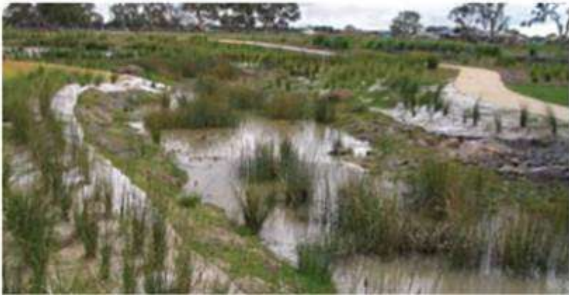
Plate 27: Example of retention basins to be used at Armstrong Creek.
