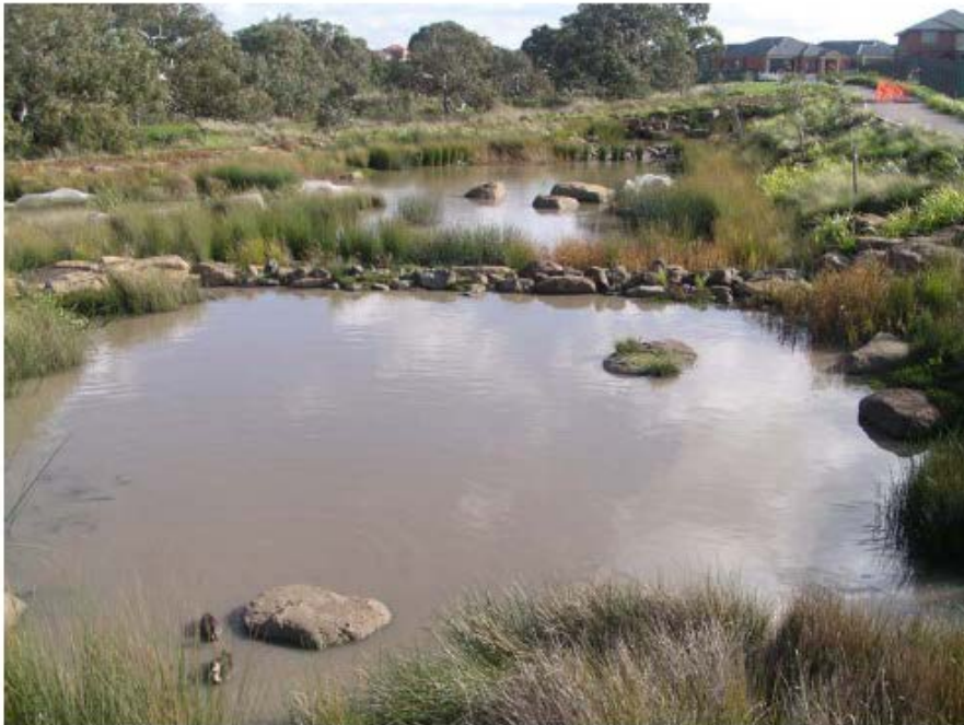
Examples of constructed wetland edges at 3:1 average slope to flanking pedestrian/bike trail (Delfin Lend Lease at Malcolm Creek, Craigieburn)
