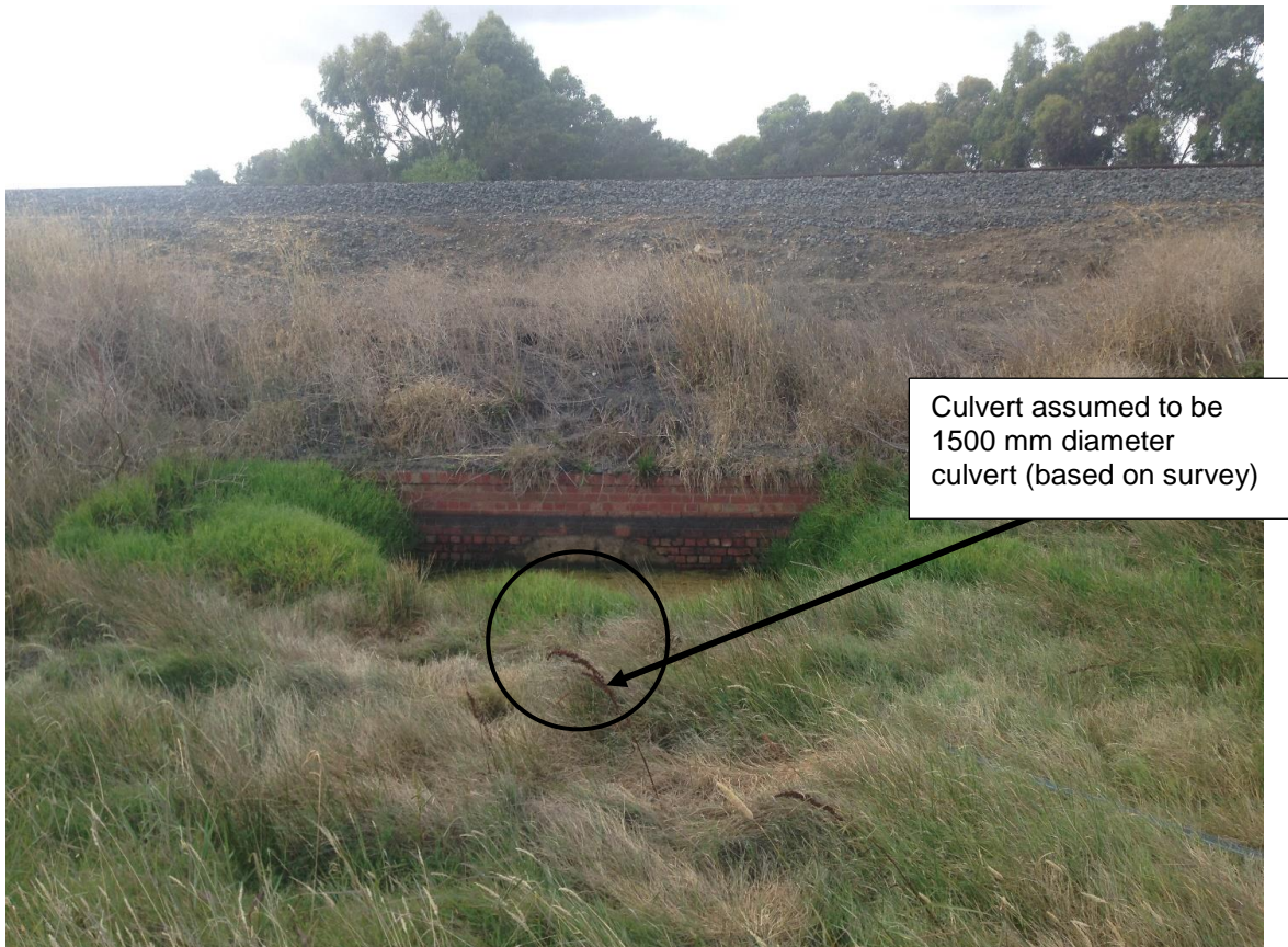
FIGURE 2-2 RAILWAY CULVERT LOCATED DOWNSTREAM OF THE SITE
