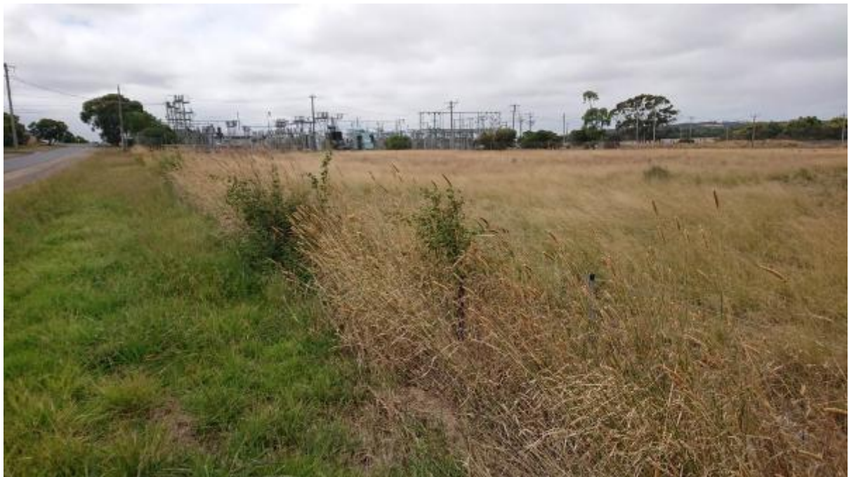
Photograph 2 Looking east toward adjacent substation
