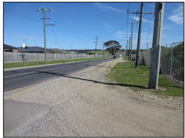
Figure 6: Ghazepore Road – view south
