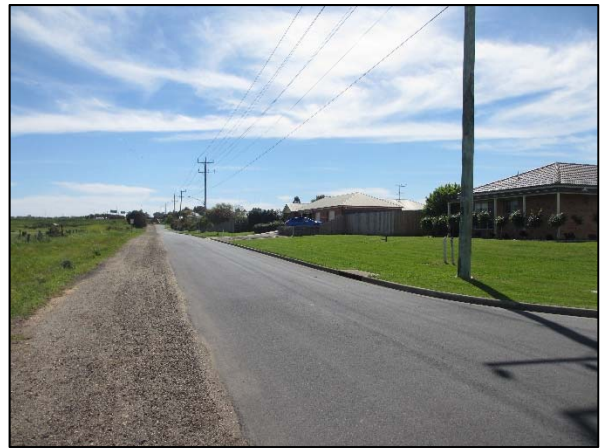
Figure 4: Hams Road – view west
