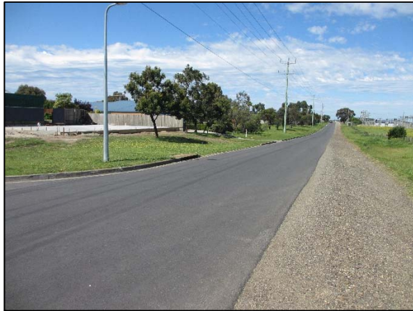
Figure 3: Hams Road – view east
