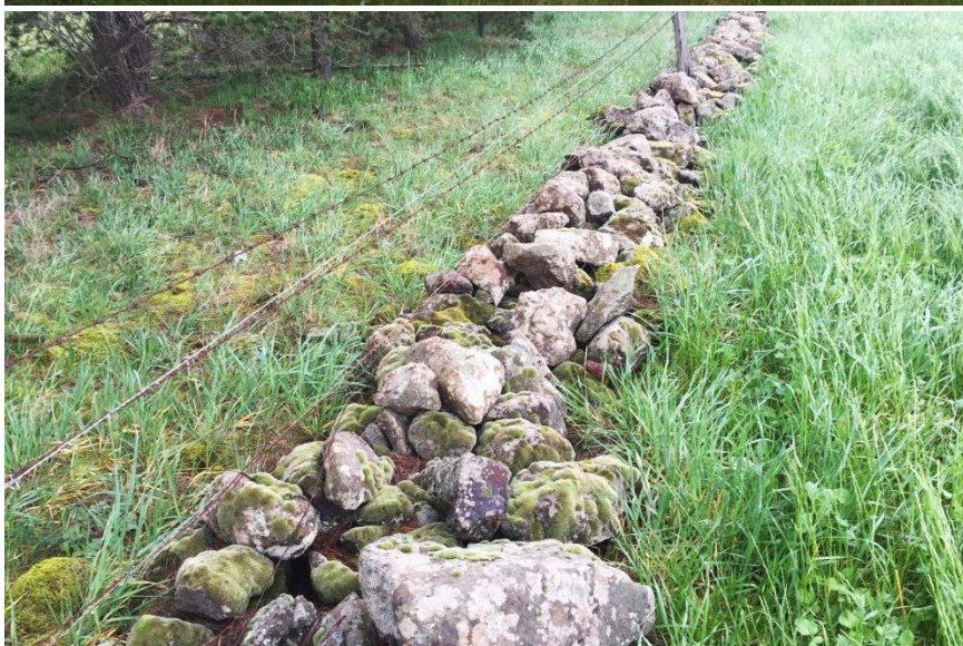
Plate 3: A more typical section of composite dry stone wall on the northern side of Elcho Road
