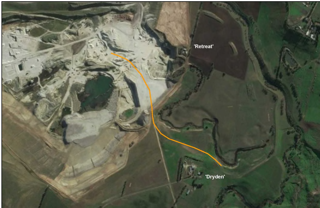
Figure 10: Aerial image showing the approximate route of the private railway tunnel
