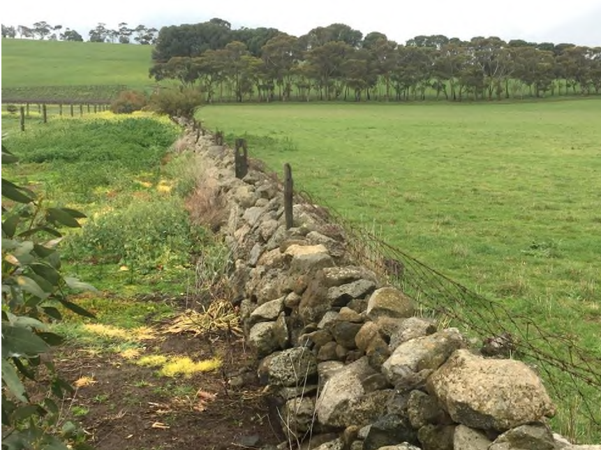
Plate 9: A section of dry stone wall south of Batesford township forming the northern boundary of Lynnburn (HO42)
