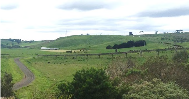
Plate 1: Remnant section of elevated conveyor between Geelong Ring Road and Moorabool River
