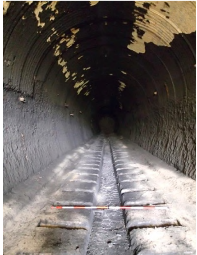
Figure 22: Tunnel interior in 2014 (Hewitt 2014: 36)
