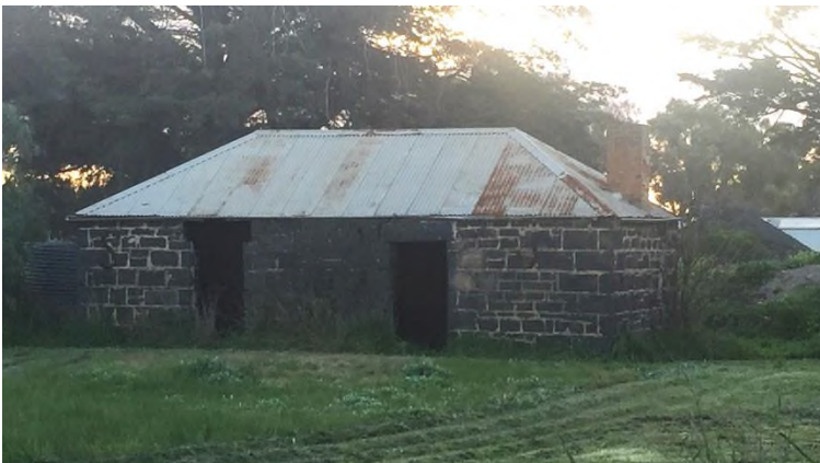
Plate 4: Ruins of the former Junction/Keens Hotel, Fyansford
