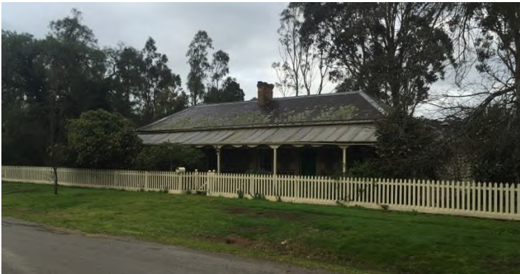
Plate 2: 'Innisfail', Cross Street, Batesford
