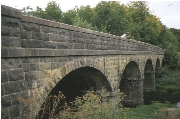
Figure 17: Bridge over Moorabool River, Batesford
