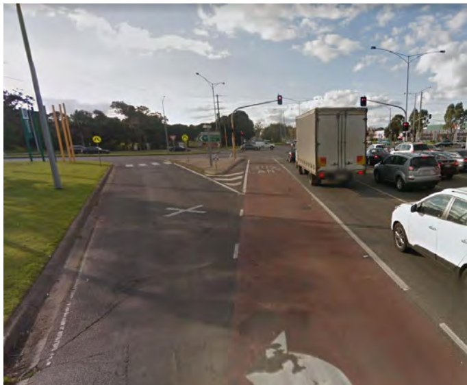
(Springvale Road / Lower Dandenong Road Intersection, Keysborough)
