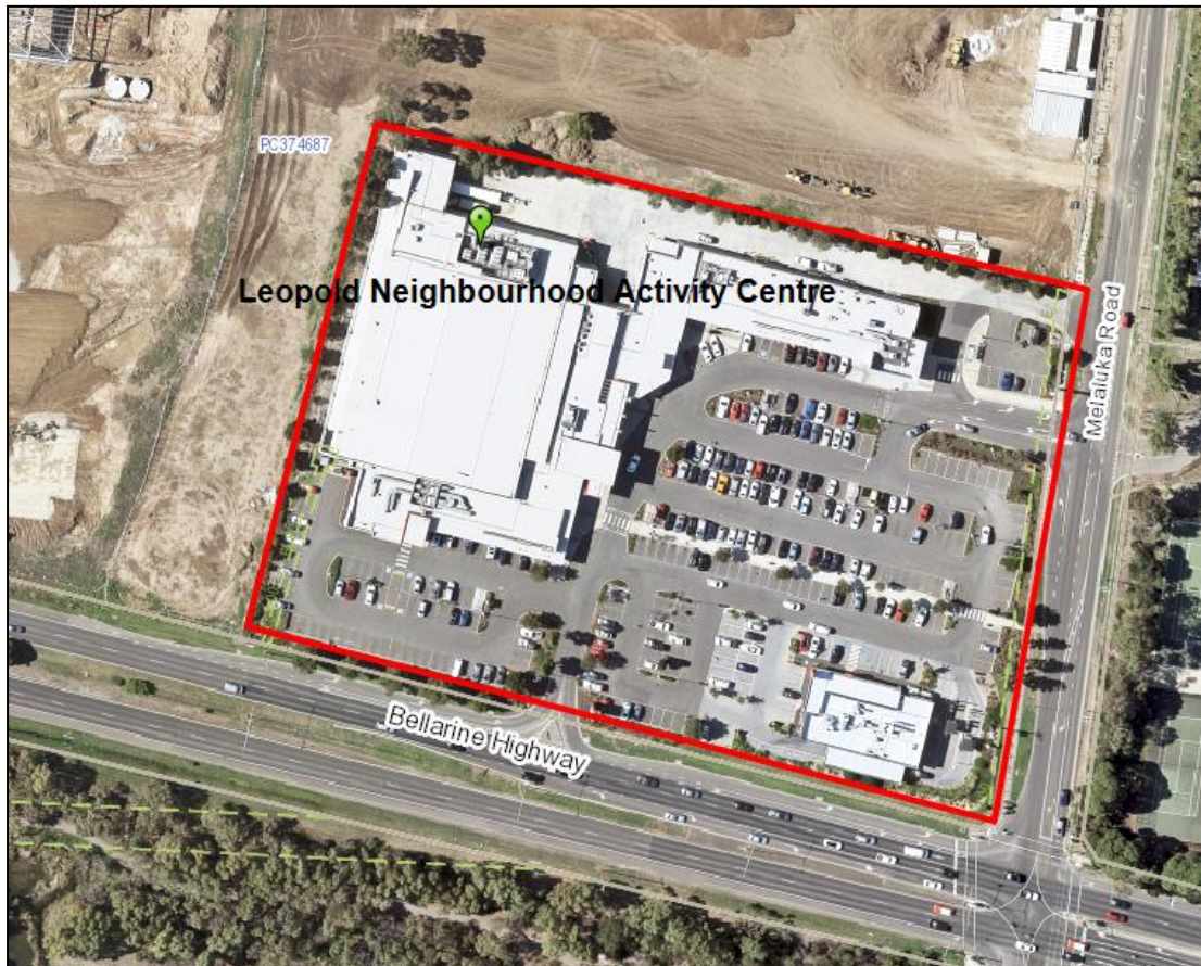
Leopold Neighbourhood Activity Centre (Full line supermarket, associated speciality retail and car parking)
