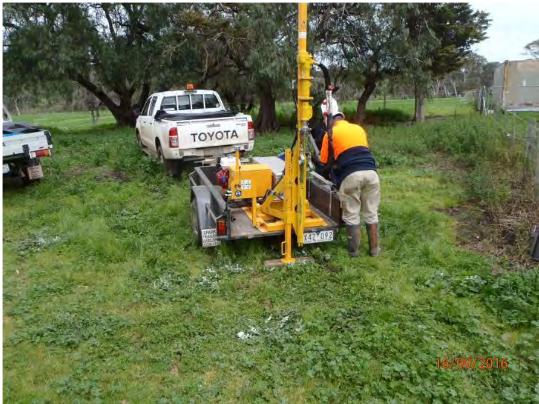
Photo 1 : BH 1 location trailer mounted push tube rig.
