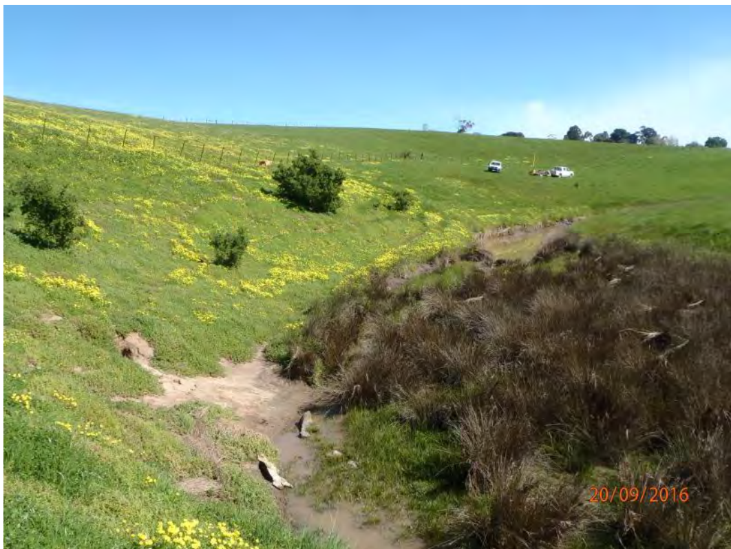
Photo 6 : Cowies Creek with exposed soil at tight bends
