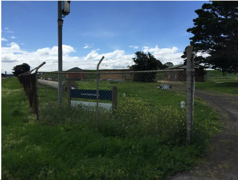
Visual assessment at BH26 – entrance to Lovely Banks Basins
