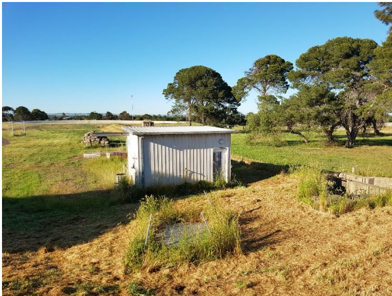
Visual assessment at BH26 – storage shed and drainage infrastructure
