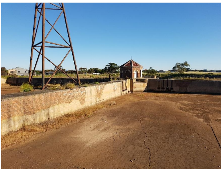
Visual assessment at BH26 – decommissioned storage basin
