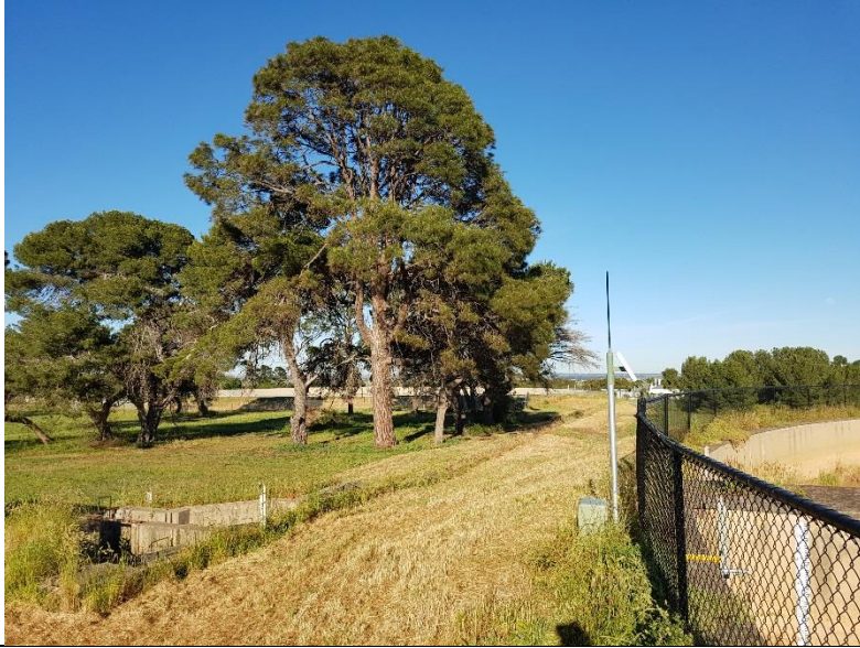
Visual assessment at BH26 – storage basin, subsurface drains and site coverage
