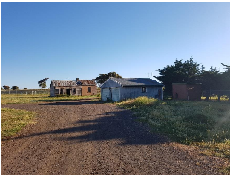
Visual assessment at BH26 – existing buildings in the south eastern area
