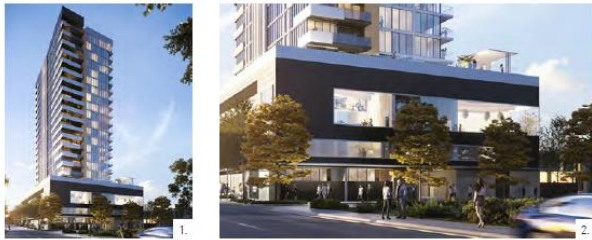
Figure 100 18-20 Cavendish Street, Geelong (PA16/00116) 1. East Elevation – Cavendish St 2. Active Frontage
