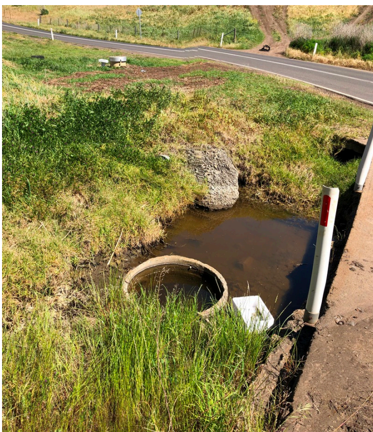
Figure 2-12 Cowies Creek downstream side of Bluestone Bridge Road
