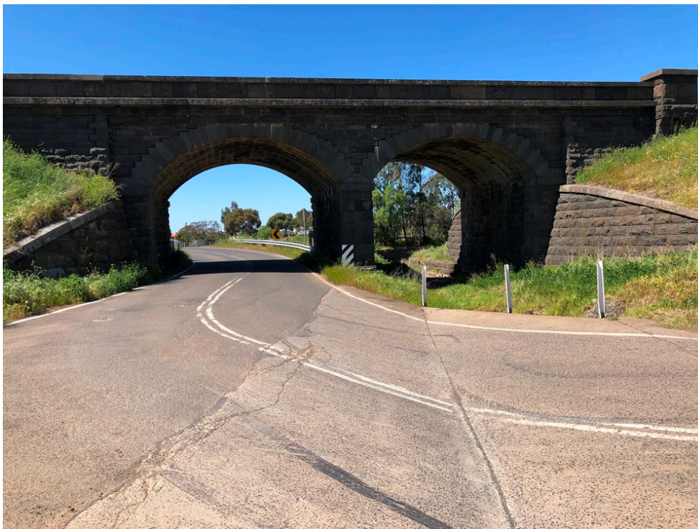
Figure 2-13 Cowies Creek – looking downstream at Bluestone Bridge Road
