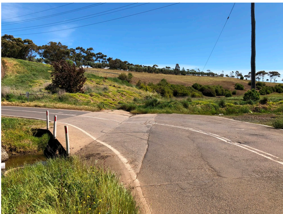
Figure 2-14 Cowies Creek – looking upstream at Bluestone Bridge Road
