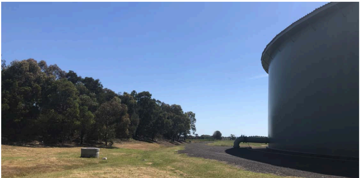
Figure 7-22 Existing planted mound to southern boundary of water tank, looking west
