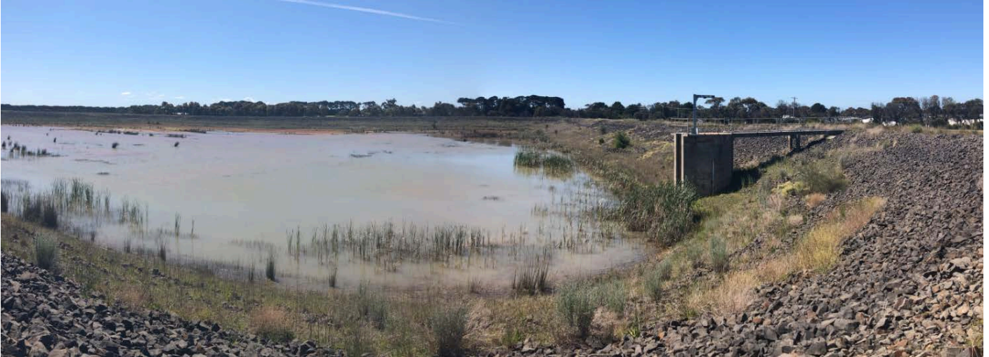
Figure 7-19 View North Across Above Ground Reservoir
