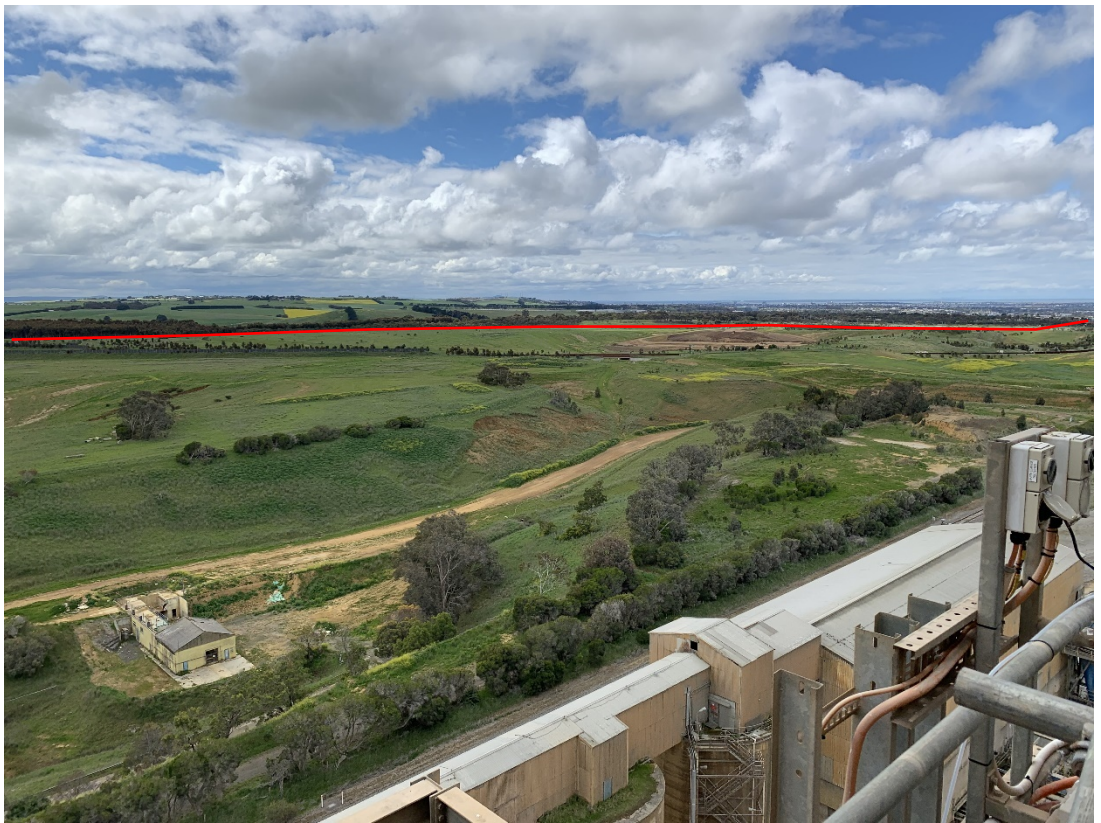
Figure 8 - View looking north over that part of the land to the north of the railway
