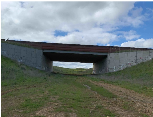
Figure 40 – Underpass under the freeway
