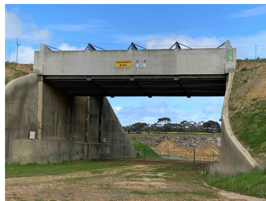
Figure 41 - Underpass beneath railway
