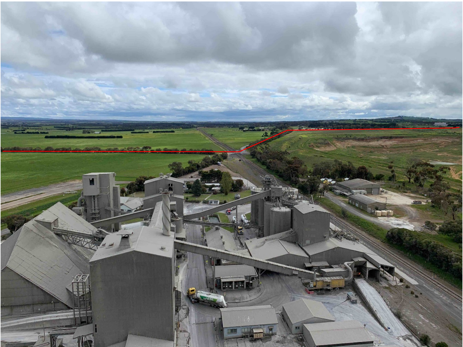
Figure 7 - View over clinker grinding facility looking west along the railway line
