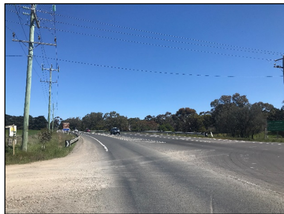
Figure 8: Anglesea Road (view south)
