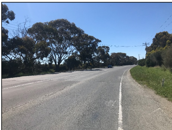
Figure 7: Anglesea Road (view north)
