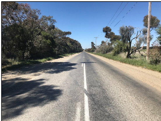
Figure 5: Reservoir Road (view east)
