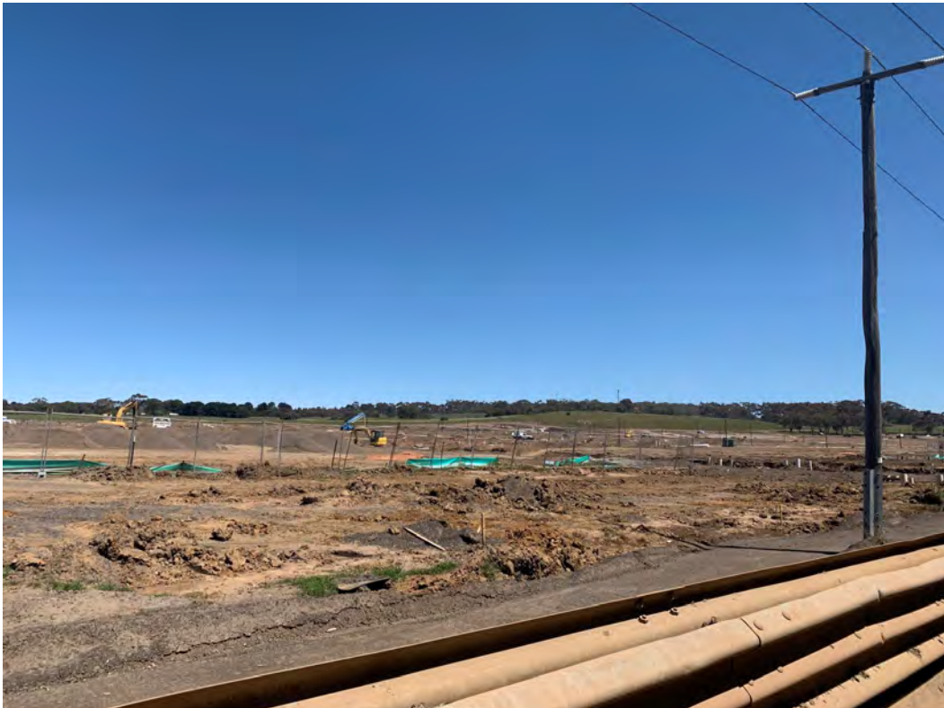
Figure 16: View towards Mt Duneed from Whites Road
