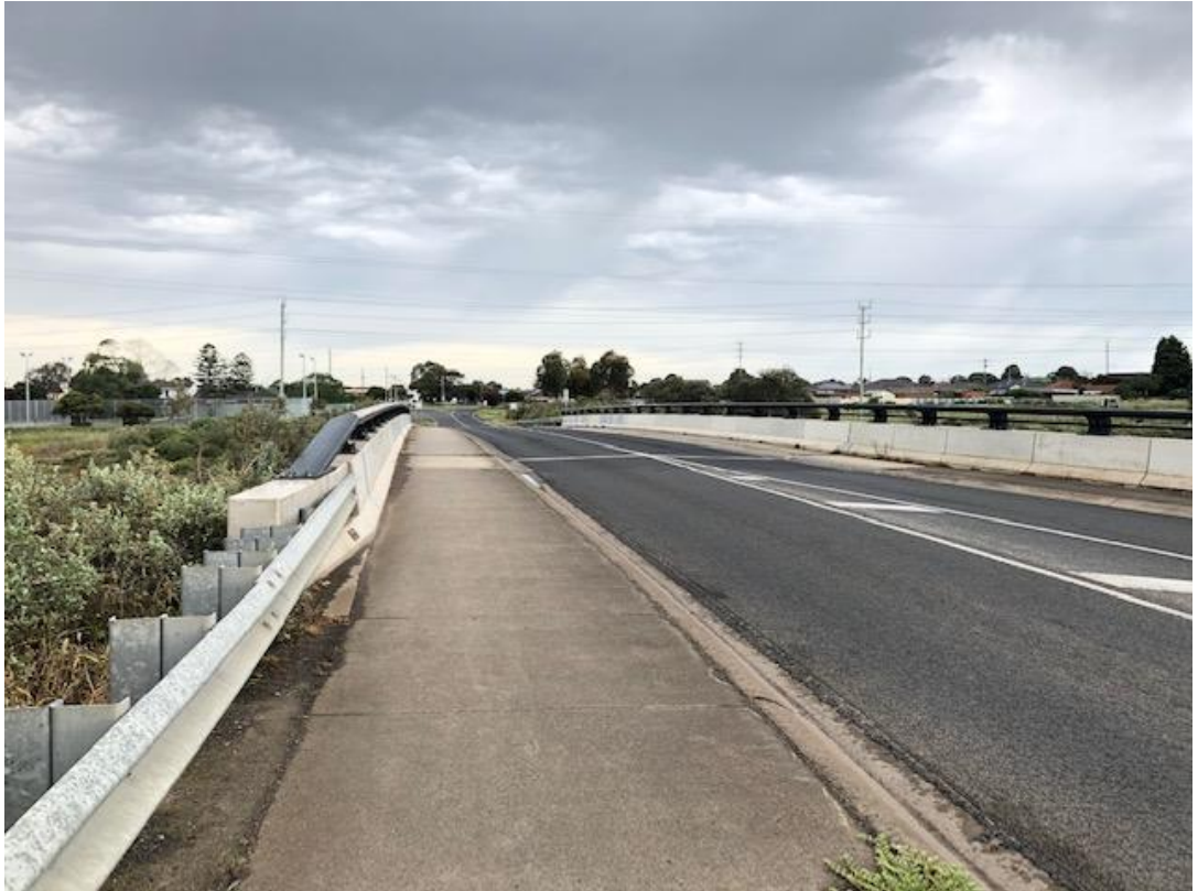
Figure 5.1 – Creamery Road Bridge over Geelong Ring Road – Looking East
