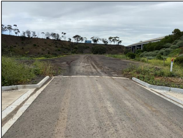
Figure 3-5 End of Sealed Road, facing southwest
