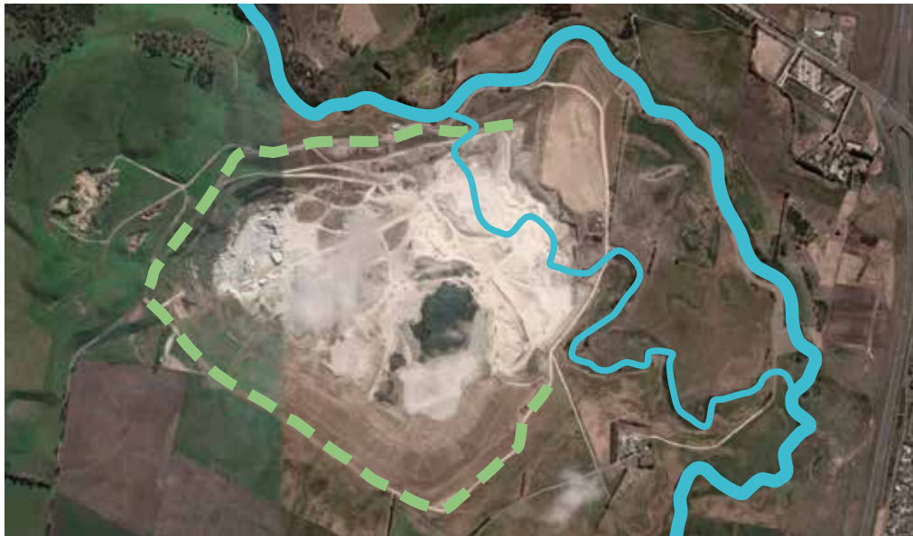
Figure 2 - 2018 ■ Extent of the rehabilitated quarry face (2018) — Original Moorabool River — Moorabool River Concrete Lined Diversion
