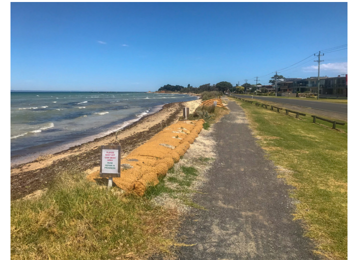
Dune repair works on The Esplanade foreshore in St Leonards
