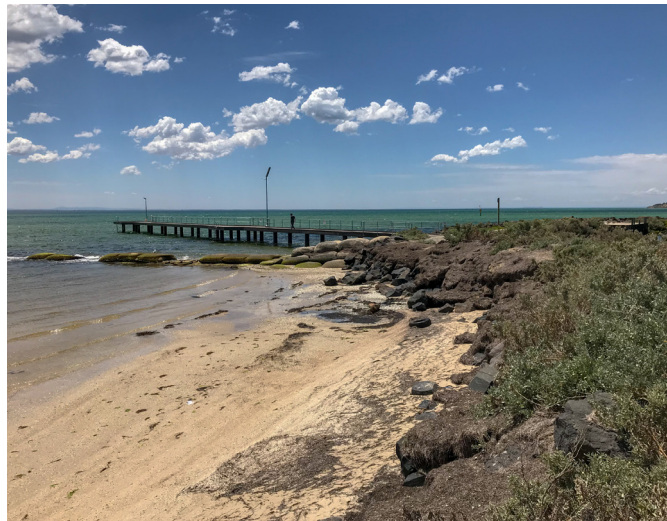
Sandbag groyne and rock revetment works at Clifton Springs
