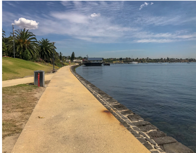
Existing bluestone sea wall along the Geelong Waterfront
