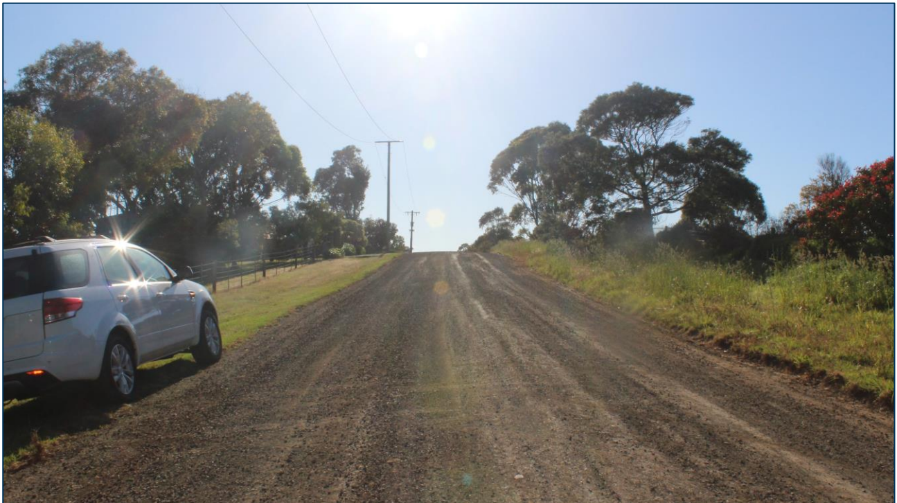
Figure 2-6 Thomas Street, looking east from Jetty Road
