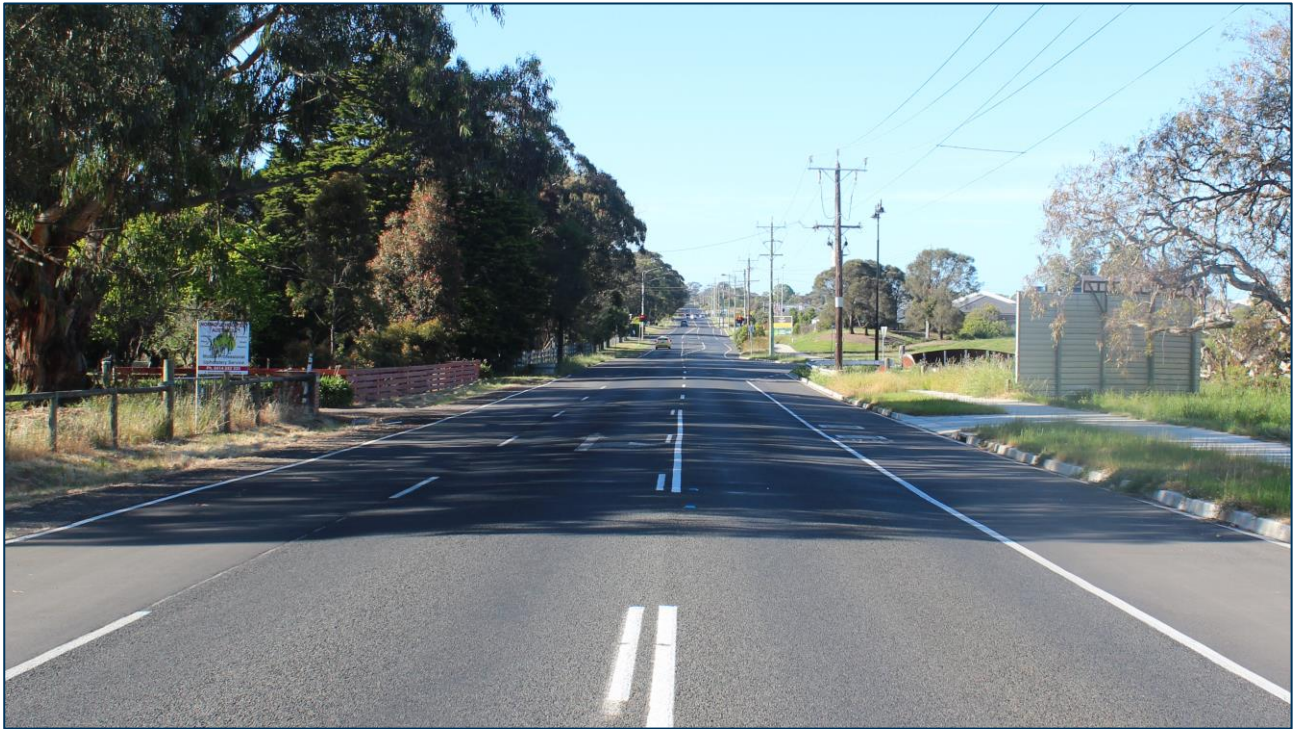
Figure 2-3 Jetty Road, looking north adjacent to subject site
