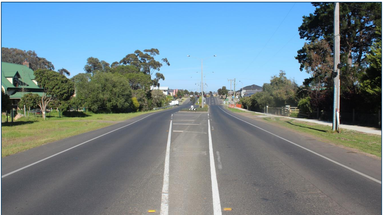
Figure 2-5 Wyndham Street, looking west adjacent to subject site
