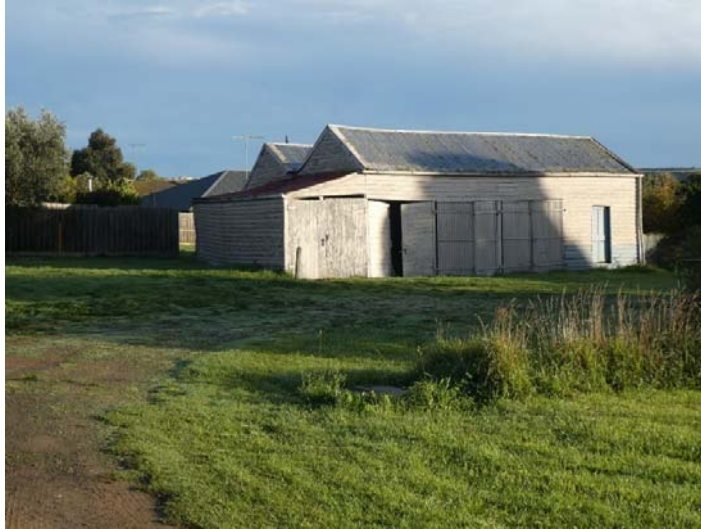
Outbuilding, south elevation, 2020. Source: David Scott, City of Greater Geelong.
