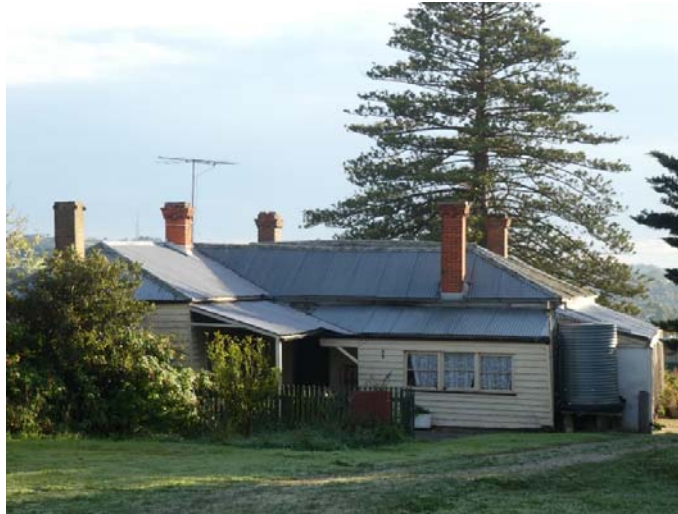
Claremont Homestead, south (rear) elevation, 2020. Source: David Scott, City of Greater Geelong.
