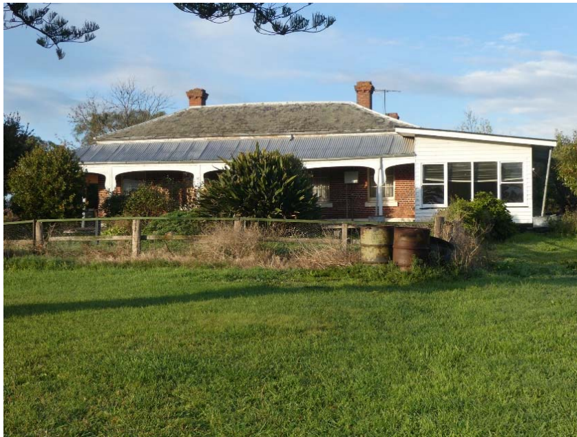
Claremont Homestead, north elevation, 2020. Source: David Scott, City of Greater Geelong.
