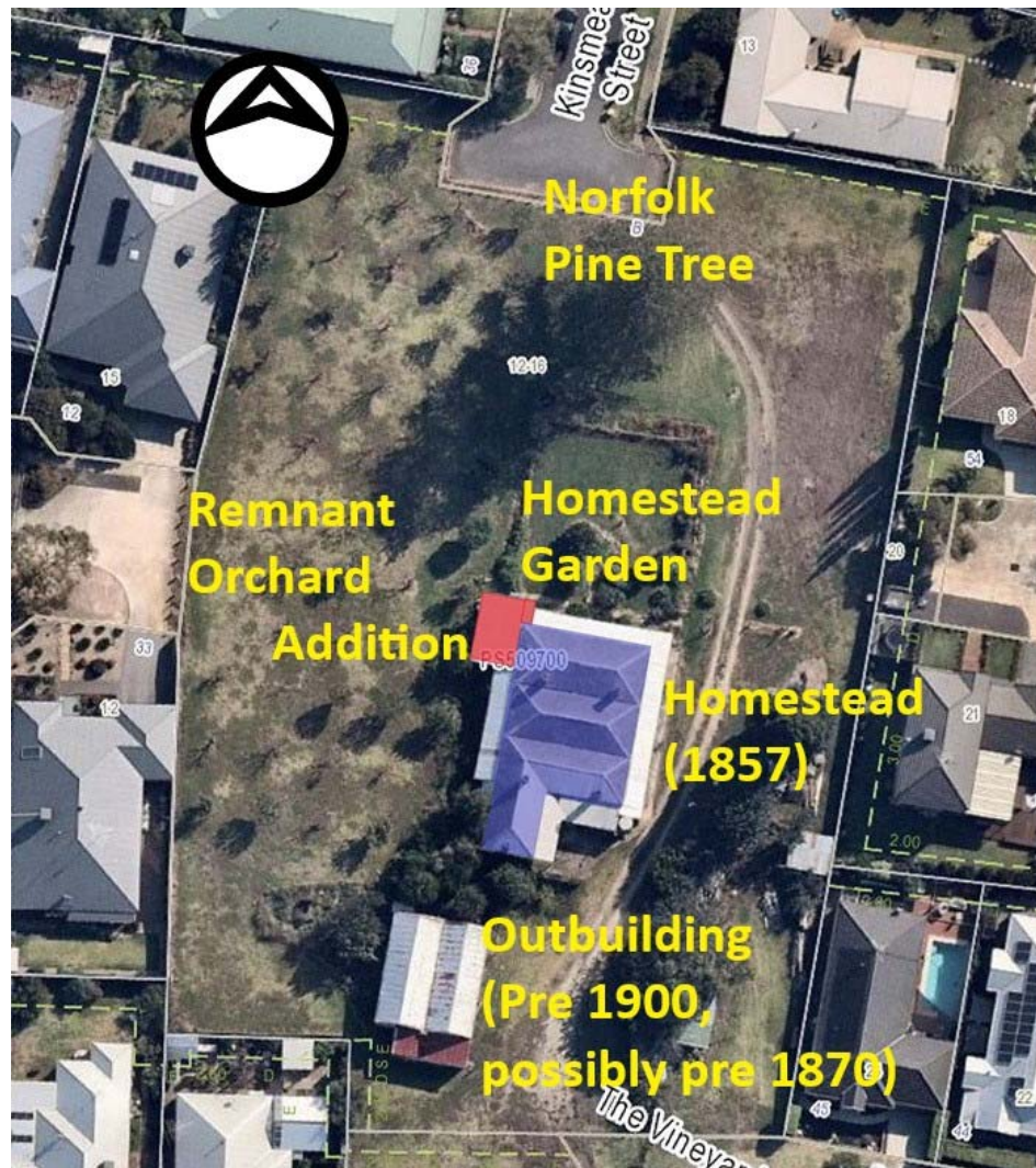
Aerial image of Claremont Homestead showing the locations and provenance of the buildings, and the landscape elements. Source: NearMap, City of Greater Geelong.
