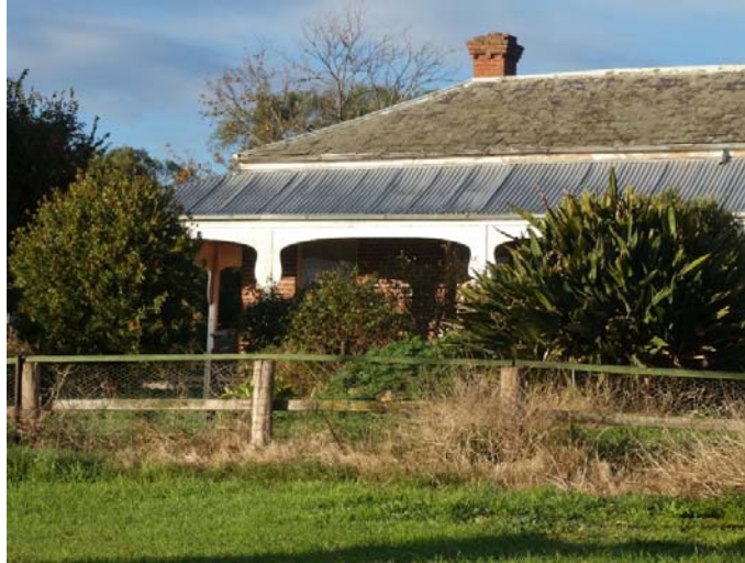
Claremont Homestead, chimney, roof & verandah detail, north elevation, 2020. Source: David Scott, City of Greater Geelong.
