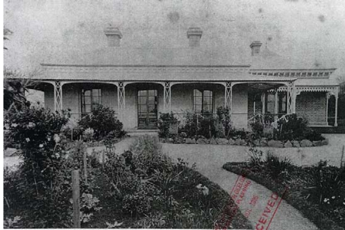
Kent Cottage, n.d. [c.1900]. Source: City of Greater Geelong.
