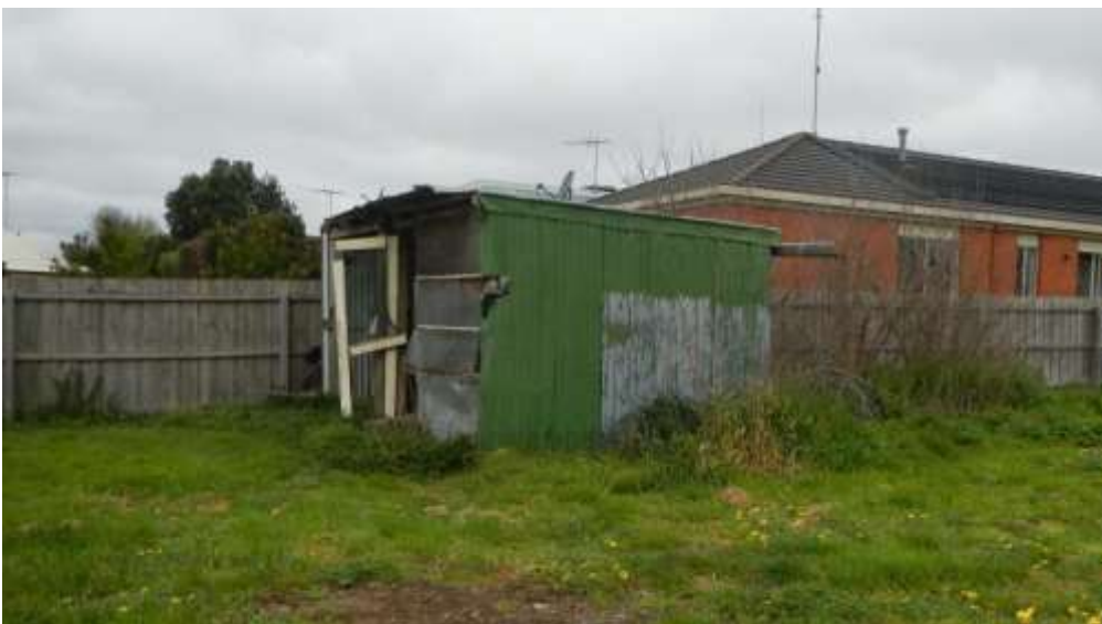
Figure 5 Shed on eastern boundary
