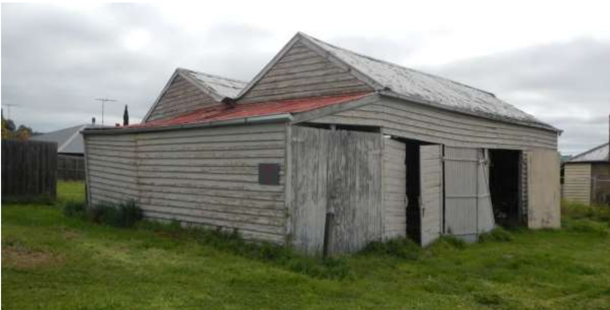
Figure 4 Large outbuilding to the south of the homestead
