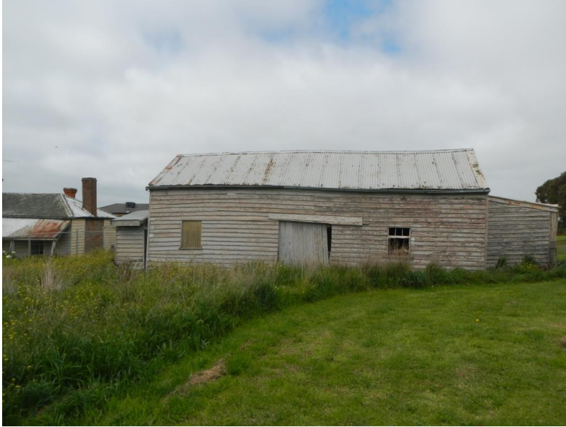
Figure 6 The west elevation of the detached double gabled timber weatherboard outbuilding.
