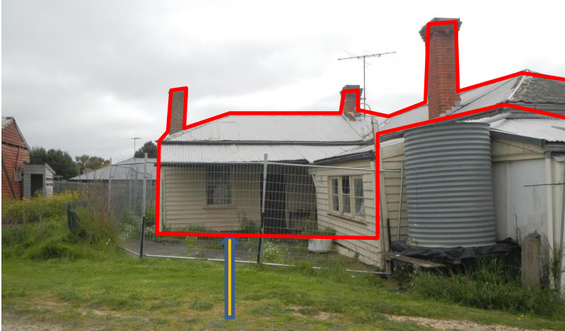
Figure 10 The existing kitchen (arrowed). Note that the kitchen walls remain behind the additions which are only included here to indicate this (See also Figure 11). If 3.2 of the Design Guidelines were implemented all of this fabric could be lost. The rear hipped roofed weatherboard section is the only old kitchen. It is not clear whether or not it is the original kitchen or a later 19 th century kitchen. Nevertheless it forms a significant part of the homestead and retains its chimney and chimney breast and cooking alcove. It also contains an indoor/outdoor well on the west side.
