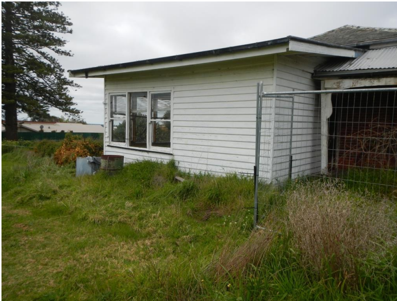
Figure 3 The post-1950s addition to the north-west corner of the front verandah.
