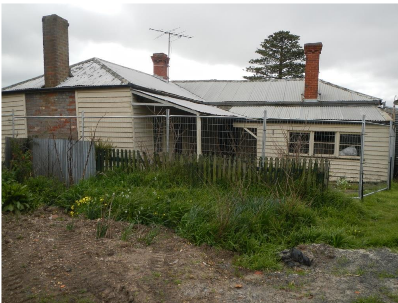
Figure 11 The south elevation of the kitchen wing.
