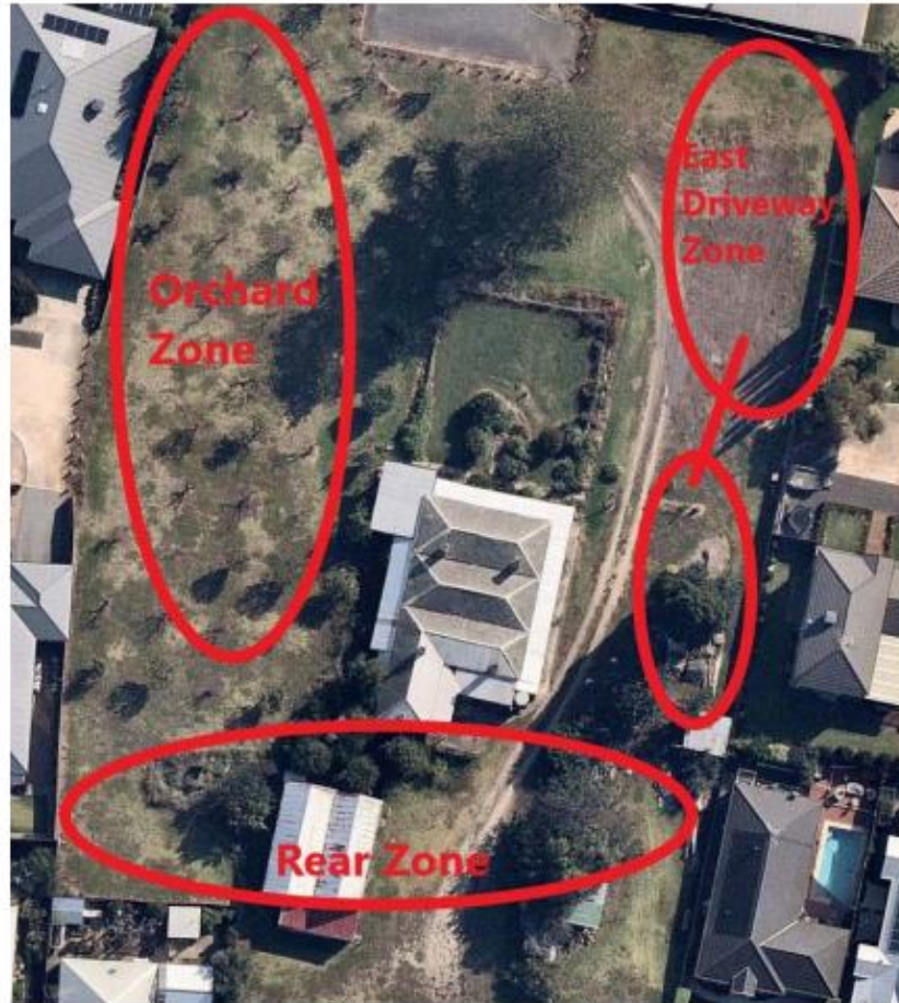
Aerial image of Claremont Homestead showing zones. Source: NearMap, City of Greater Geelong, 28 March 2020.
