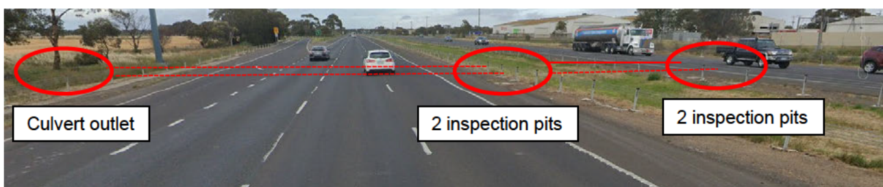
Figure 27 Location of Princess Hwy Culverts (Southern Culverts – 15 Avalon Rd, Lara)
