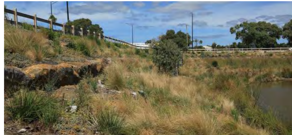
Figure 4.19 - SC Hwy/Burvilles Rd wetland eastern 1:2.5 - 1:3 vegetated batters
