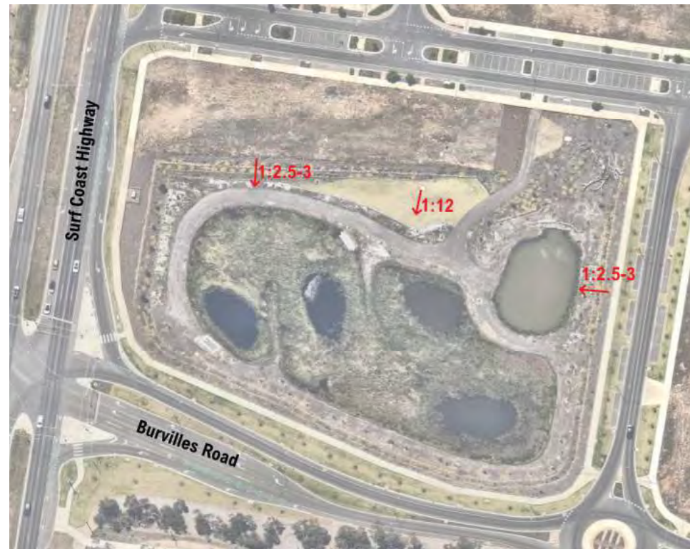
Figure 4.17 - Aerial photo of Surf Coast Hwy/Burvilles Rd wetland with batter slopes
