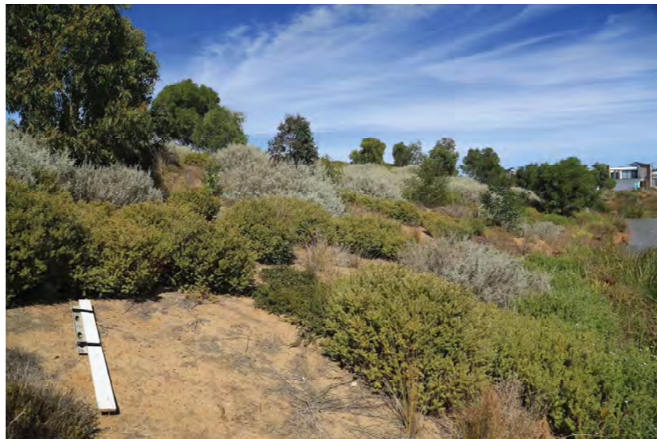
Figure 4.13 - Eastern batter slopes - 1:4
