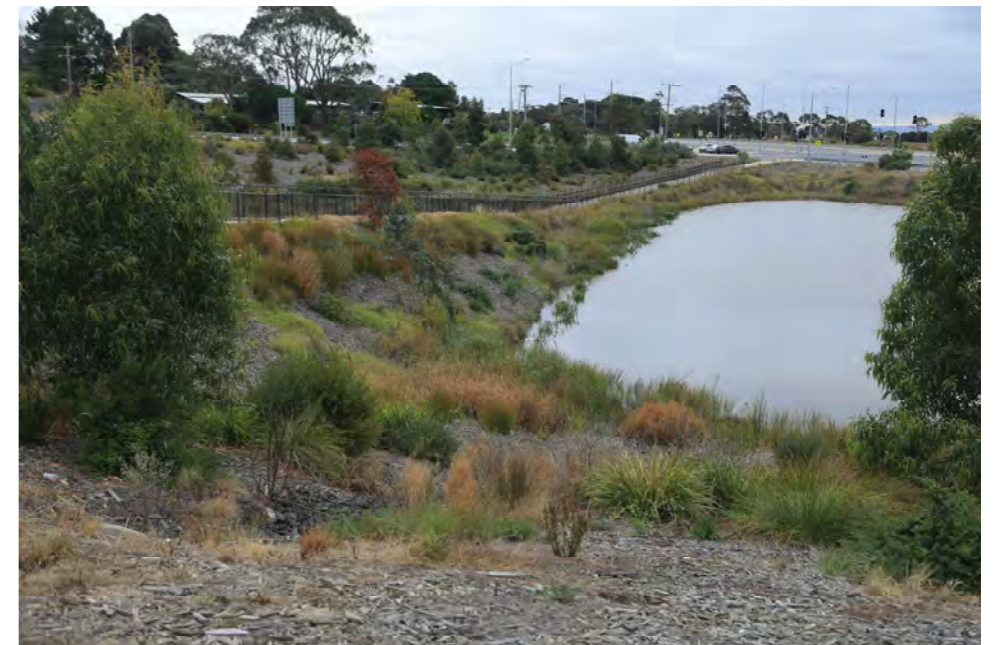
Figure 4.37 - North-eastern batter slopes from the shared pathway
