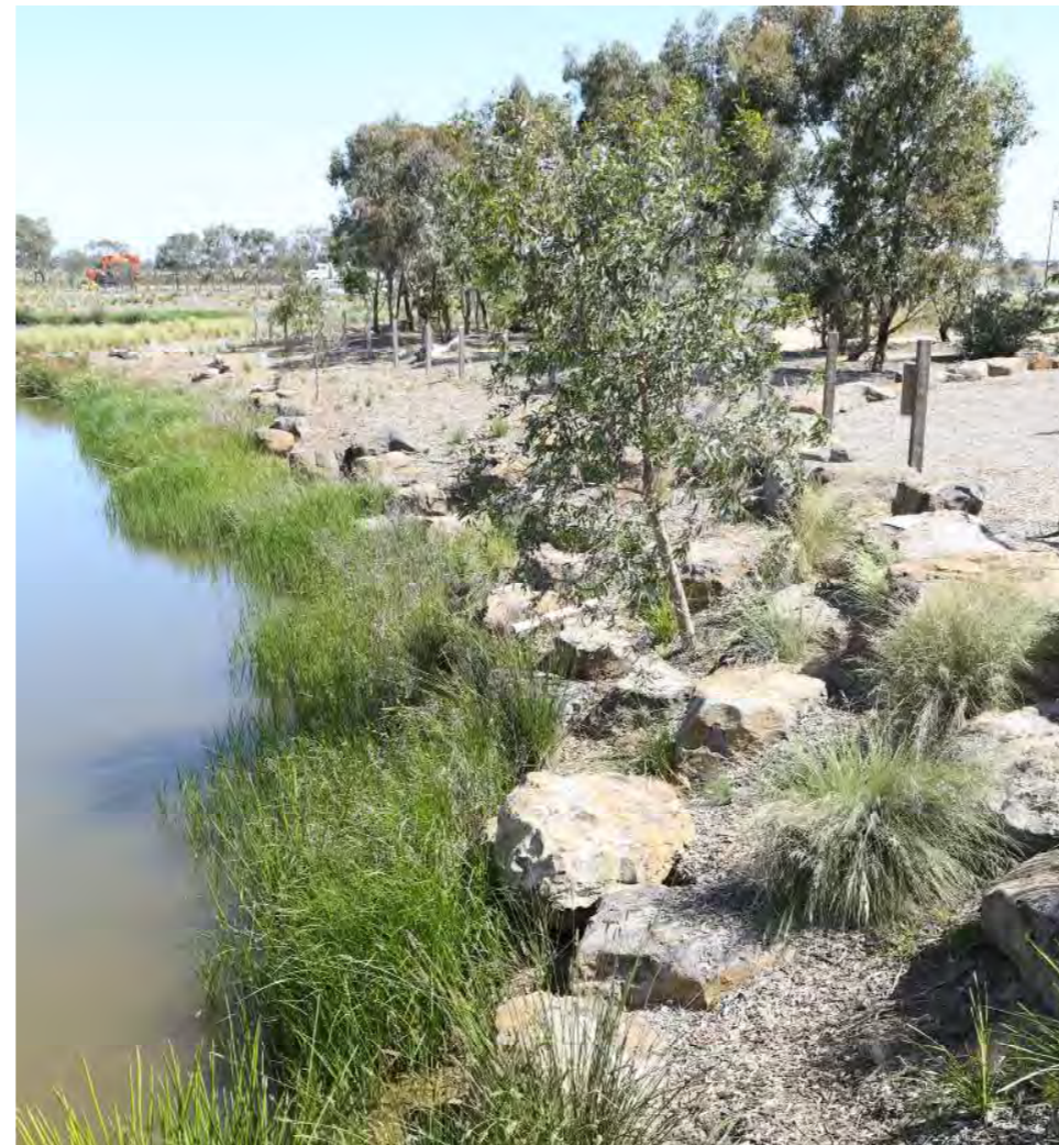
Figure 4.25 - Warralily rock stabilised and vegetated batter (2014)
