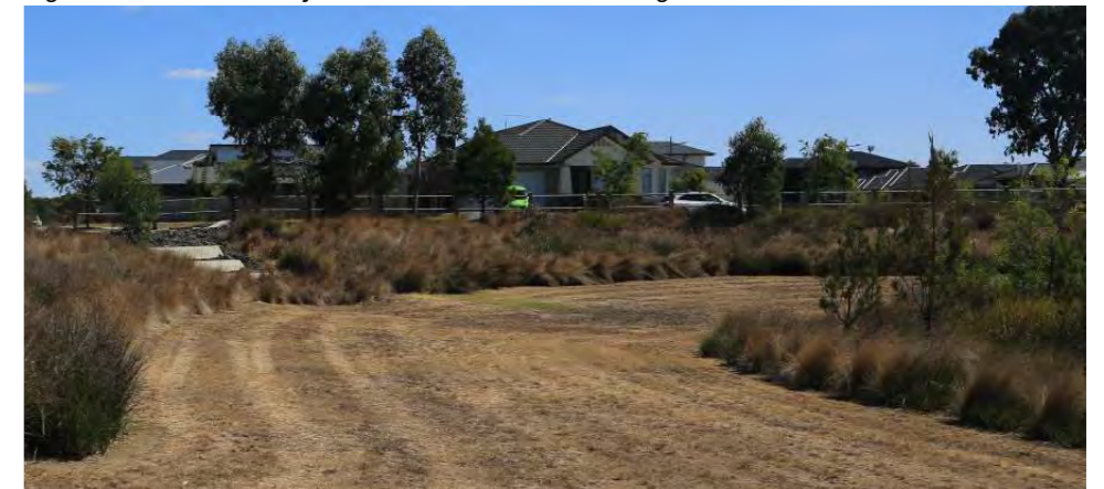
Figure 4.23 - Sanctuary Blvd wetland western 1:3.5 - 1:4 vegetated batter
