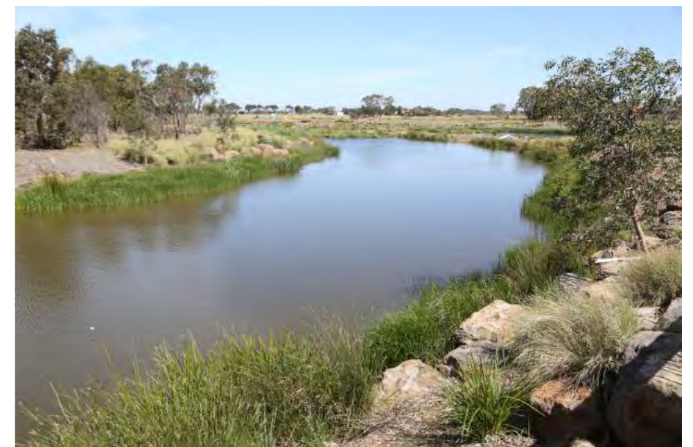
Figure 4.26 - Warralily rock stabilised and vegetated batter (2014)
