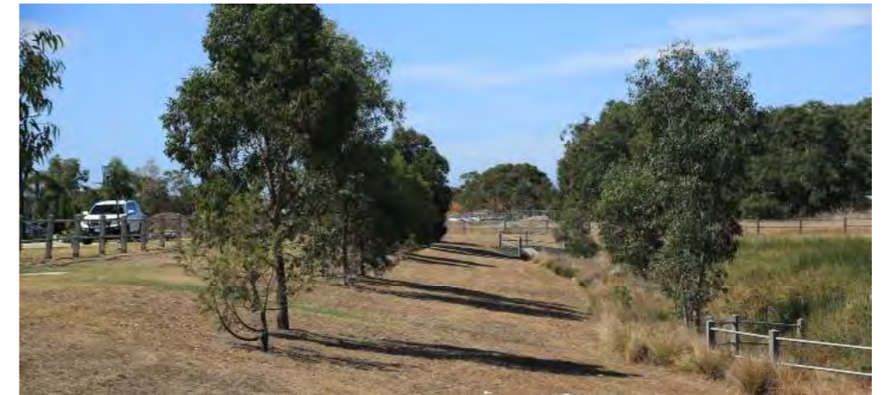
Figure 4.22 - Sanctuary Blvd wetland northern 1:6 grassed batter
