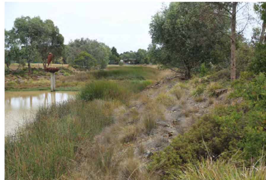
Figure 4.28 - Estuary Blvd rock stabilised and vegetated batter
