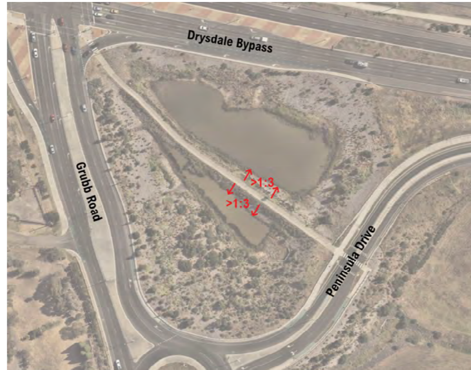
Figure 4.34 - Aerial photo of Peninsula Drive wetland with batter slopes
