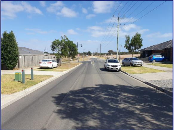
Figure 16: Coriyule Rd (East of Tivoli Dr) - View West
