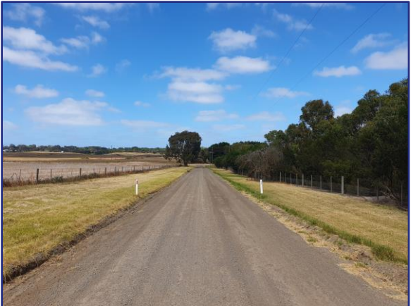
Figure 20: McDermotts Rd - View South
