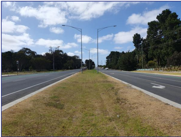
Figure 9: Portarlington Rd - View East
