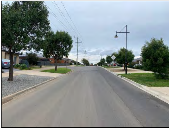
Figure 6: Coriyule Road (east of Tivoli Drive) - view east
