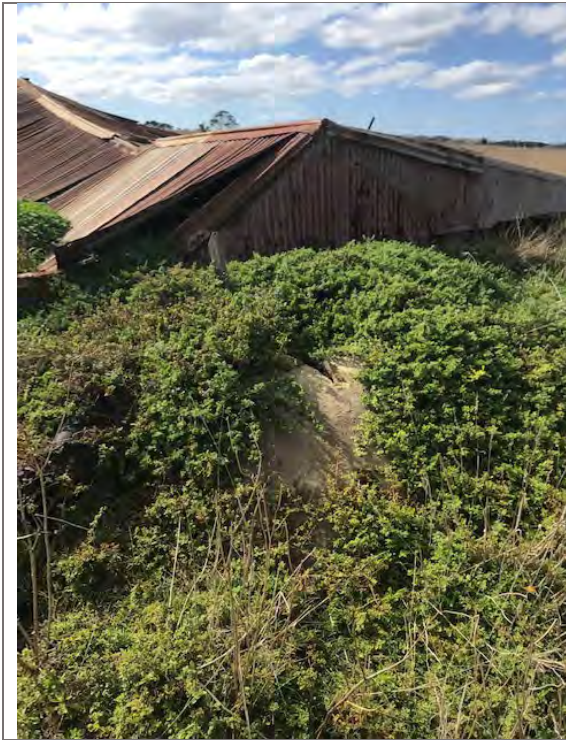
Photo 1: Former Shed and top of in-ground water tank
